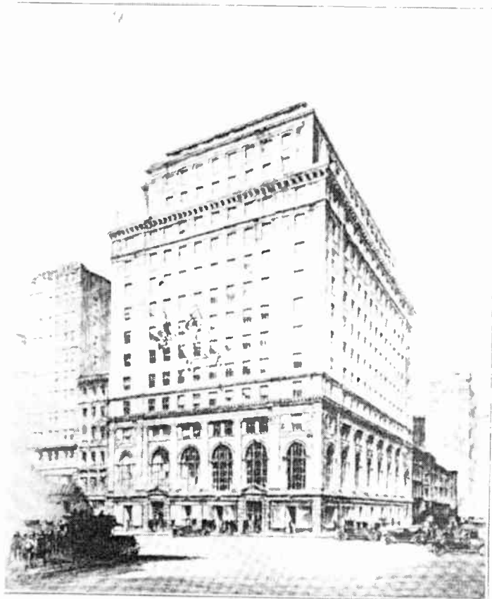
FIG. 5.—The new building to be occupied by the National Broadcasting Company in New York in which the most elaborate broadcasting studio facilities will be installed for supplying its increasing number of station subscribers and commercial clients.
