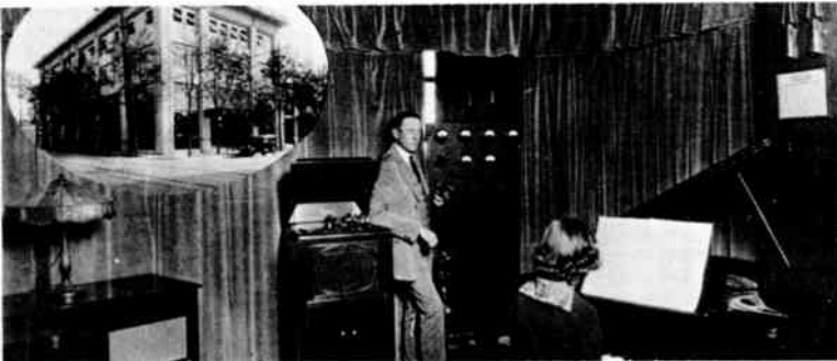
First studio and transmitter of KFI, Los Angeles
