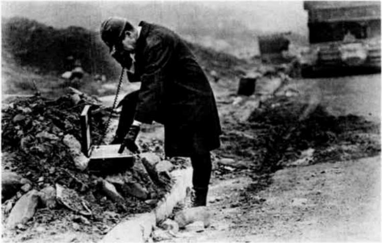
*A portable telephone at a construction site saves installation of temporary phone lines.*
