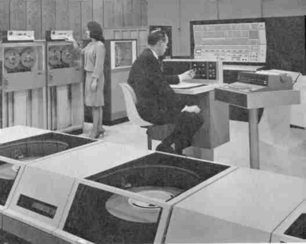
*Computer installation with disk packs in foreground and tape drives at left.*
