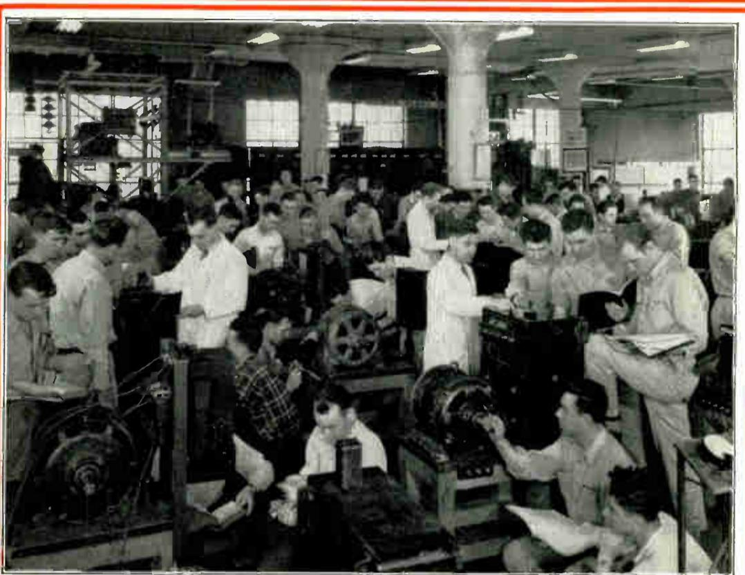
Another view of a section of our A. C. department showing students working on a wide variety of A. C. motors and control equipment. You learn how to inspect, connect up, test and repair many types of A. C. machines. Notice the modern fluorescent lighting units mounted on the ceiling. Our entire building is equipped with this modern type of lighting.
