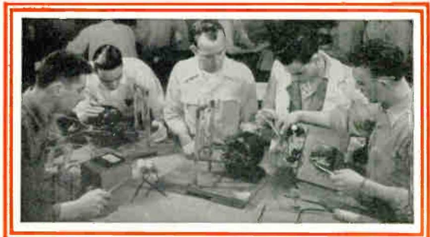
These students are making a Lock-torque test on A. C. Motors to determine the effect on the starting torque when various size capacitors are used.
