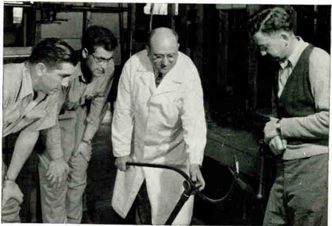
This Instructor is giving a personal demonstration on handling conduit. Most of the new and modern wiring for lights and power is run in these pipes called conduit. A practical man working in this line must know how to bend, cut and thread this conduit. These Students are getting a practical demonstration on bending conduit. This training is designed to prepare graduates for work in wiring of houses, buildings, etc.
