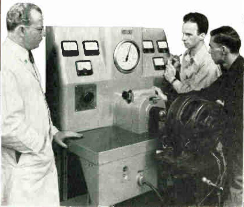
These Coyne students are testing a generator with a modern Dynamometer, a type used extensively in industry for testing A.C. and D.C. motors and generators.
