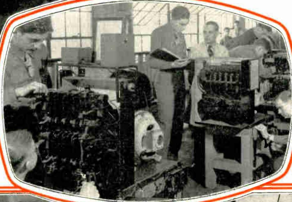
Students learning care and adjustment of automatic and remote controlled A. C. motor starters, relays, contactors, coils and other equipment in the Coyne Alternating Current Department.
