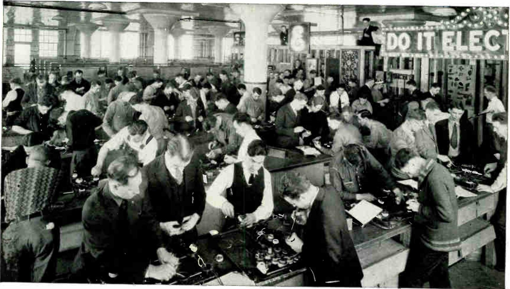
General view of a section of the electrical wiring department. Notice the large and well lighted shop. The men are wiring and testing light control circuits in their first small conduit layout, and getting real practical experience in the handling of tools and the use of various kinds of switches.
