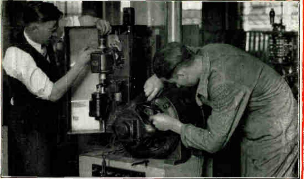
These students are checking the operation of an automatic controller and compound motor. They are making the same test and repairs they may be called upon to make in the field.
