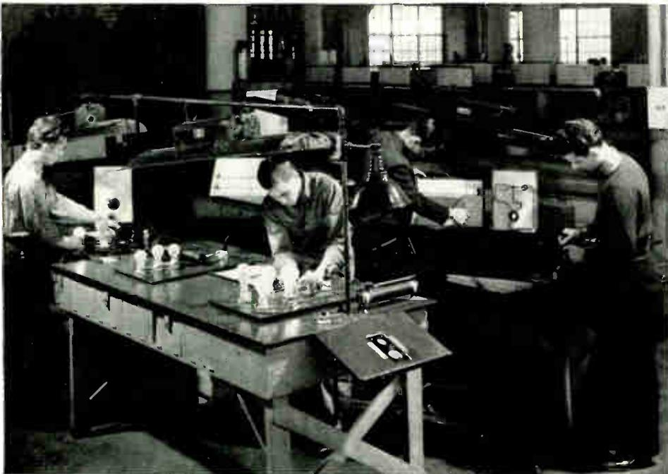
Here you see students testing neon signs, fluorescent and mercury vapor lights, such as used in many plants and factories, and lighting control units. Such practical instruction gives you a good understanding of how to use and apply modern lighting equipment.
