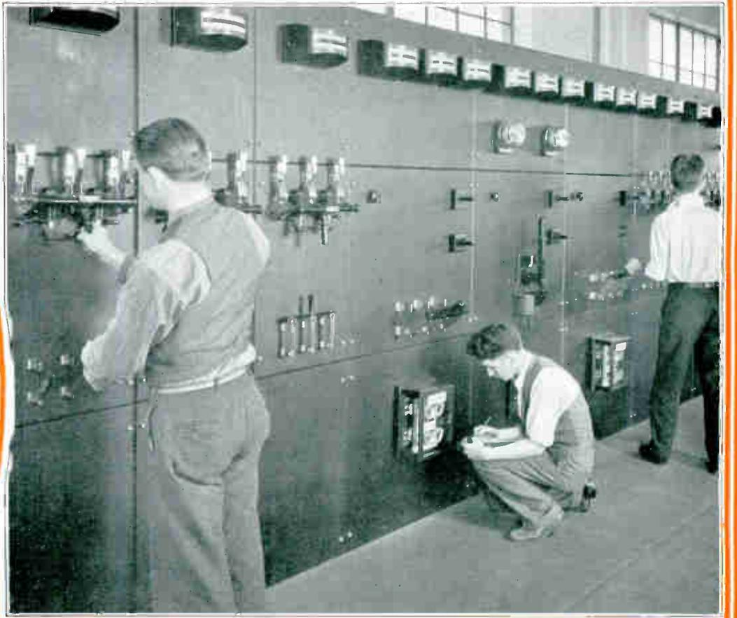
And these men are getting actual operating practice on a large A. C. switchboard. Here they learn the operation and care of meters, circuit breakers and switches, and how to synchronize and operate alternators in parallel and equalize their load. And in this way qualify for the fine positions in A. C. Power plant operating.
