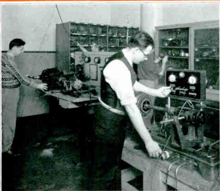
These fellows are using modern garage type test benches for giving final running tests to generators and starters they have overhauled and repaired. Your work on such equipment will help you qualify for the real jobs in this line.
