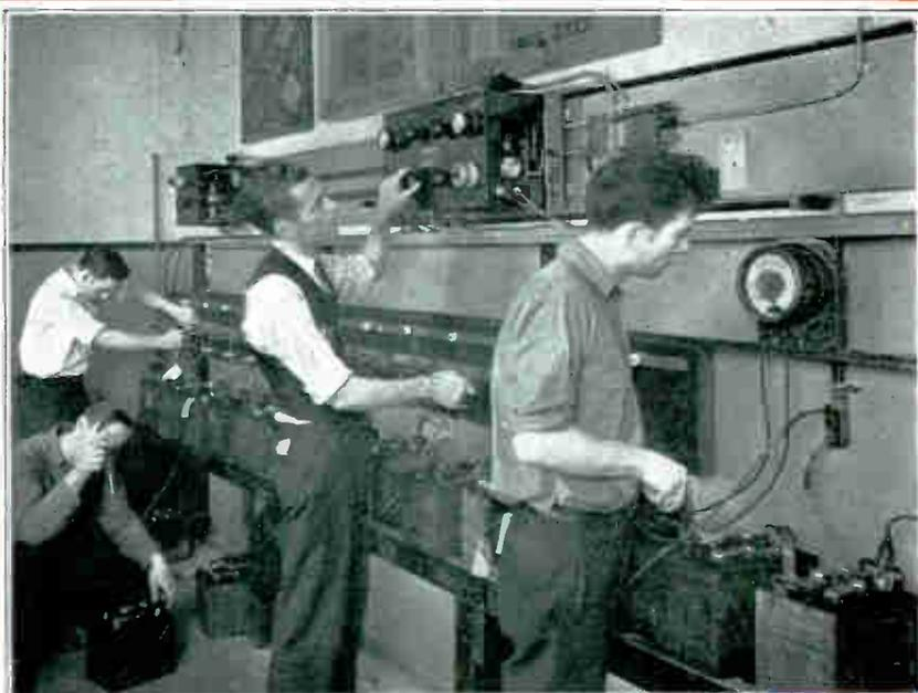
And here they are operating the charging line and equipment of the Tungar type. Both the half wave and later type full wave chargers are used here. And you see these men testing the acid, and the voltage to determine the exact condition of the batteries being charged.
