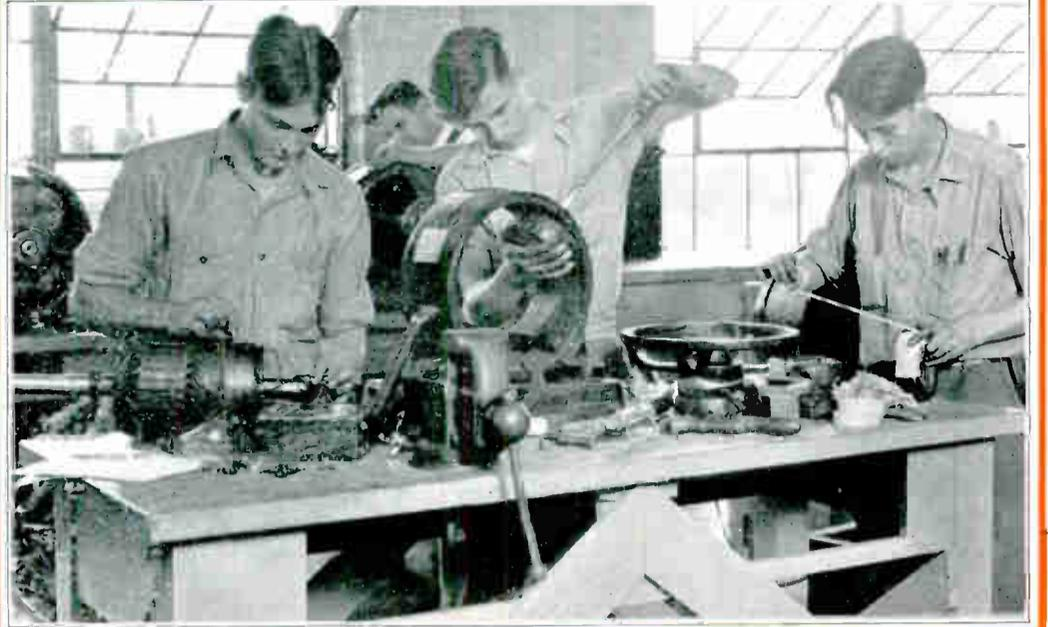
Real practical training. These fellows are completely overhauling and repairing a D. C. motor, and repairing the field coils, and the commutator and armature.
