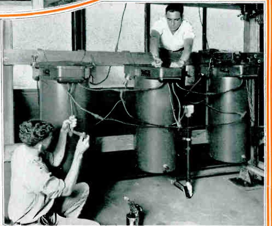
These fellows are connecting up a bank of power transformers for 3 phase operation, in the outdoor type substation in this department.
