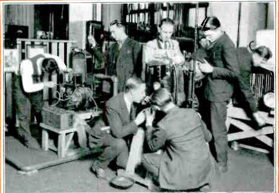
These fellows are working on a farm lighting plant. Here you will learn the care and operation of farm lighting plant equipment, and the automatic plant which starts and stops itself as lights are turned on or off. Many of our graduates are making good money selling, installing and servicing such plants.
