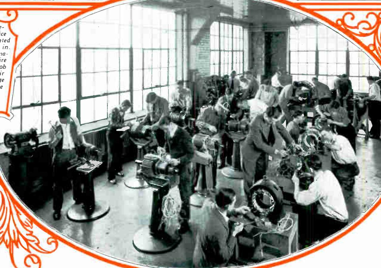
These fellows have finished their first small winding and here you can see them winding and testing large armatures and stators. In the background you will see men trueing up a commutator in a lathe and others winding a 200 h. p. A. C. stator. And in the foreground one of the instructors showing a student how to test his finished winding, before connecting up the leads.
