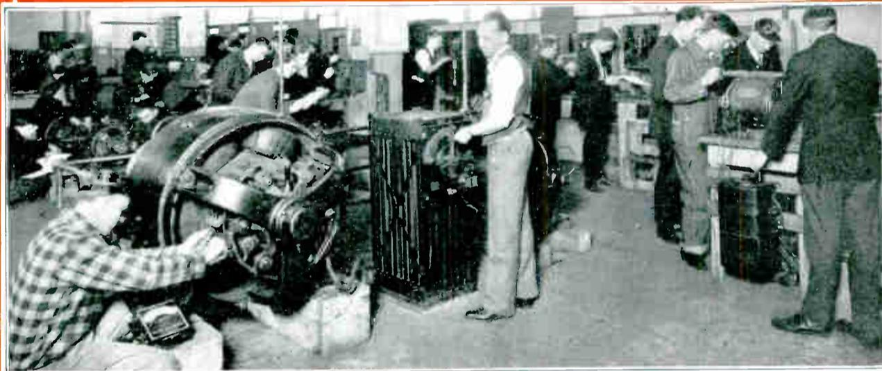
Here you see several of my students testing and operating generators. The large machine at the left, is used to make practical demonstrations of a three wire generator, and also dynamic brake tests.
