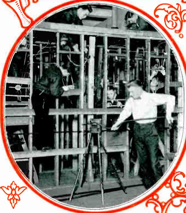
These fellows are putting in wiring in conduit, BX, and knob and tube, in the actual house frames, and learning to wire lights and switches the same as they will out on the job.
