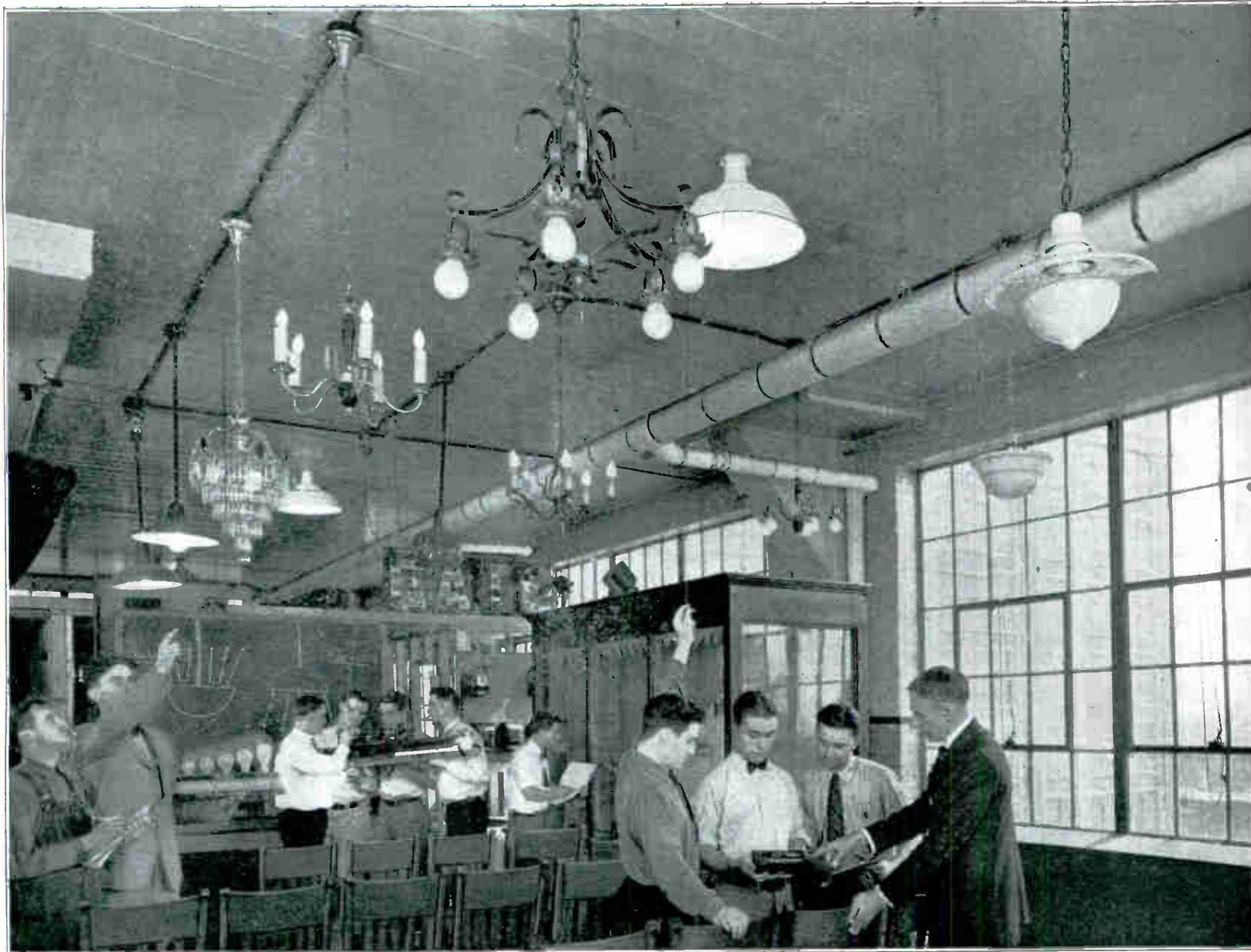
Here you see part of the illumination section, and some of the different kinds of light fixtures you work with. The instructor in the right foreground is showing students how to test the amount of light from each fixture with a "foot candle meter." You learn which type of fixture is best for home, office, or factory use.
