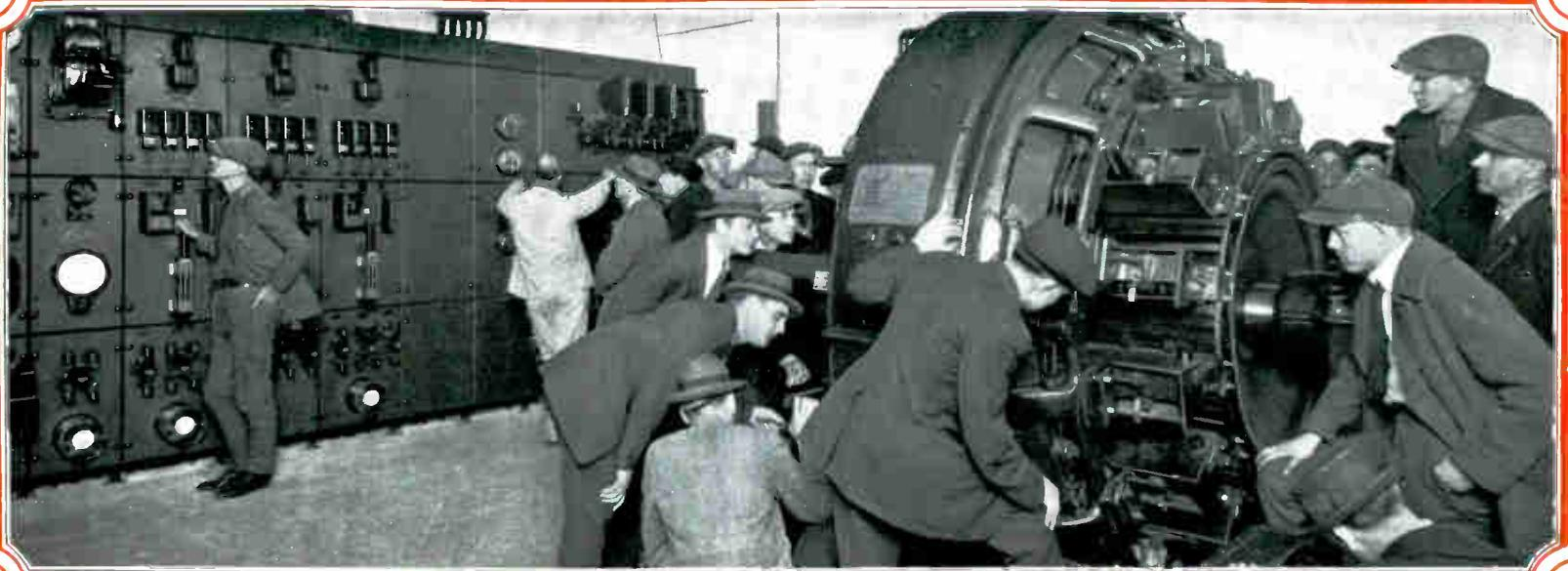
This is an automatic substation of the street railway systems, and the fellows are shown examining the 2000 K. W. converter, and switchboard. Trips to such plants as these inspire the fellows to work harder and are intensely interesting to our students.
