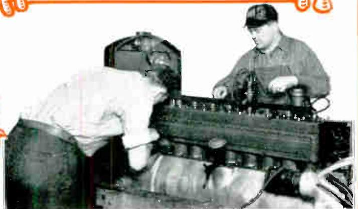
And here you see a Packard "5 cylinder in line" engine. These men are checking the firing order and connecting ignition wires to the spark plugs properly. Work on such engines as this makes you able to handle the good jobs in ignition work.
