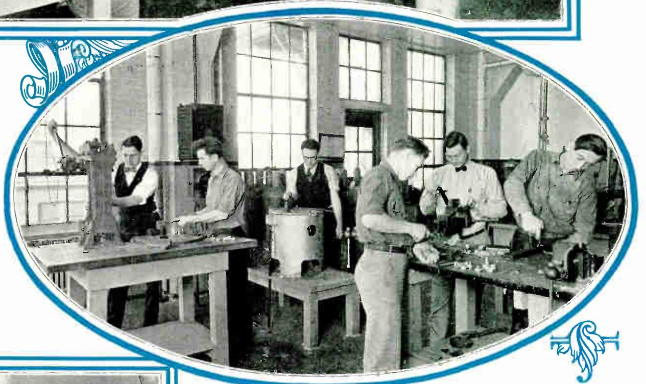
And these fellows are melting lead in a modern electric melting pot, and moulding lead posts and straps for the batteries they are building. This work gives them excellent practice with tools, and modern equipment.
