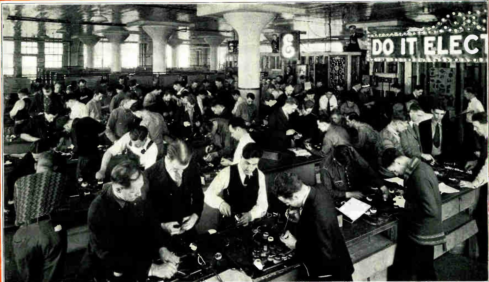
Here you see a general view of a section of my construction or wiring department. Notice the large and well lighted shop. The men in this picture are wiring and testing light control circuits in their first small conduit layout, and getting real work with the tools and different kinds of switches.
