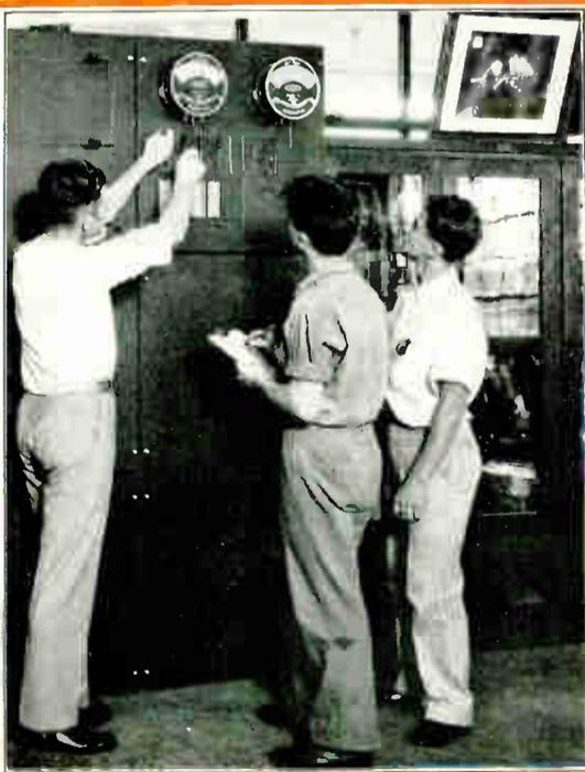
This picture shows the instructor explaining how the current flows through different resistance coils. Then he shows how this is proved out by the meters which you see on the top of the board.
