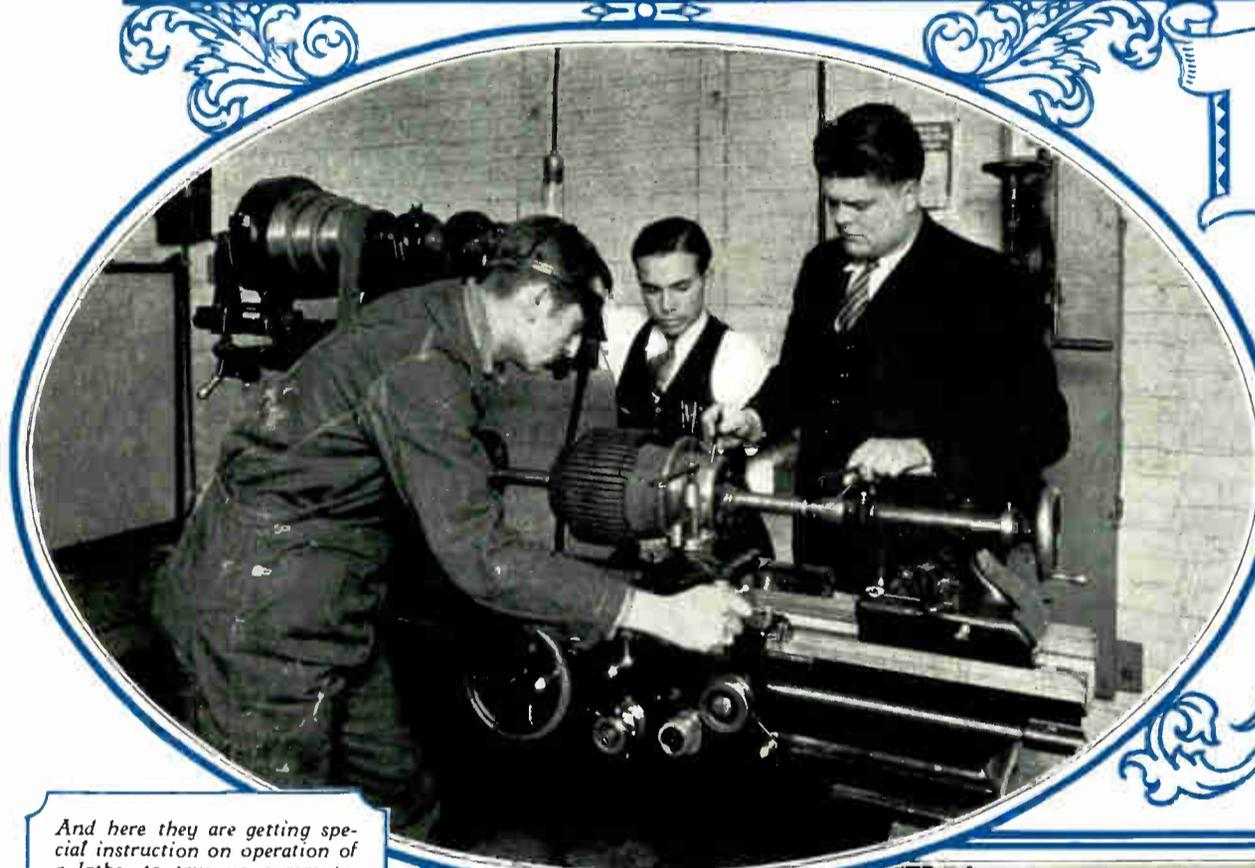
And here they are getting special instruction on operation of a lathe, to true up commutators on armatures. The instructor shows them how to grind and set the cutting tool, and how to make a nice smooth cut on the copper.
