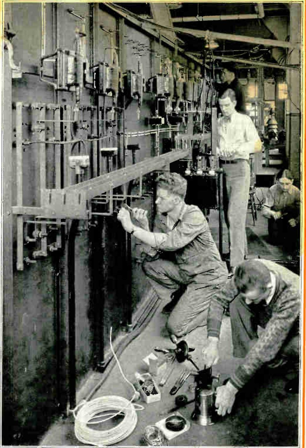
Real switchboard construction. Here you see several of my students putting additional circuits on the main A. C. switchboard. They are installing bus bars, cables and conduit, and instrument transformers. So you see how my complete training qualifies you for anything that comes up on the job.
