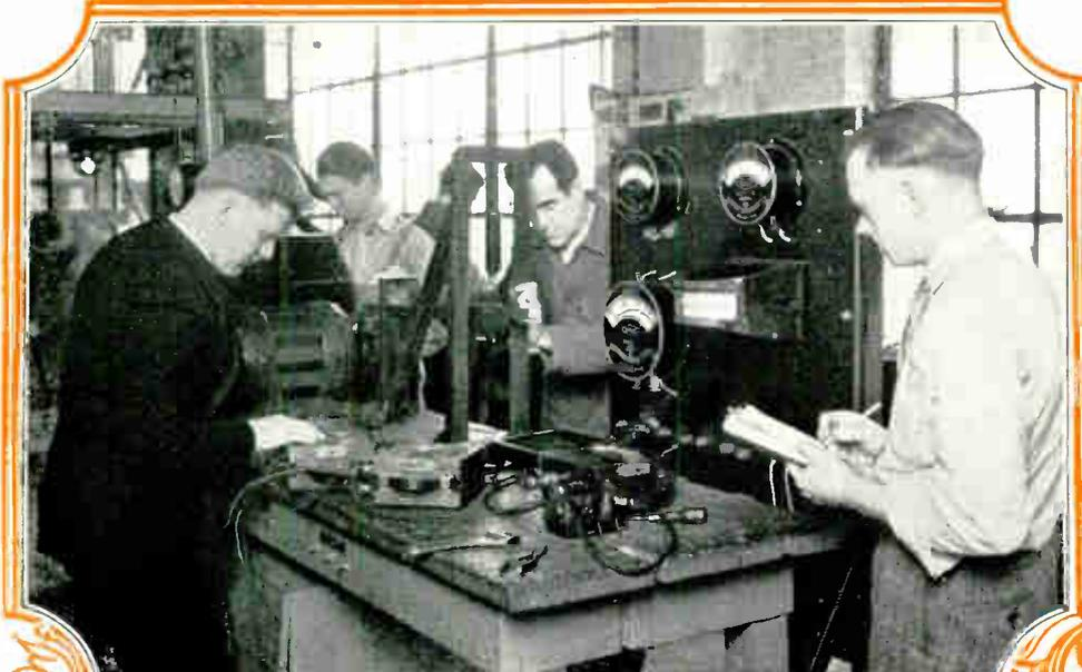
These men are testing the horsepower, efficiency, and power factor of an induction motor. All very valuable things for the practical maintenance man to know.
