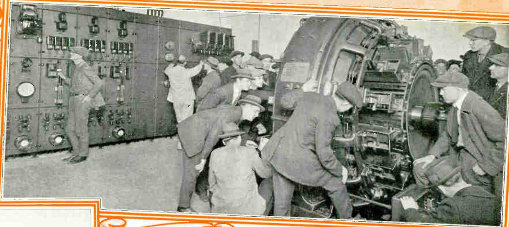
This is an automatic substation of the street railway systems, and the fellows are shown examining the 2000 K. W. converter, and switchboard. Trips to such plants as these inspire the fellows to work harder and are intensely interesting to our students.
