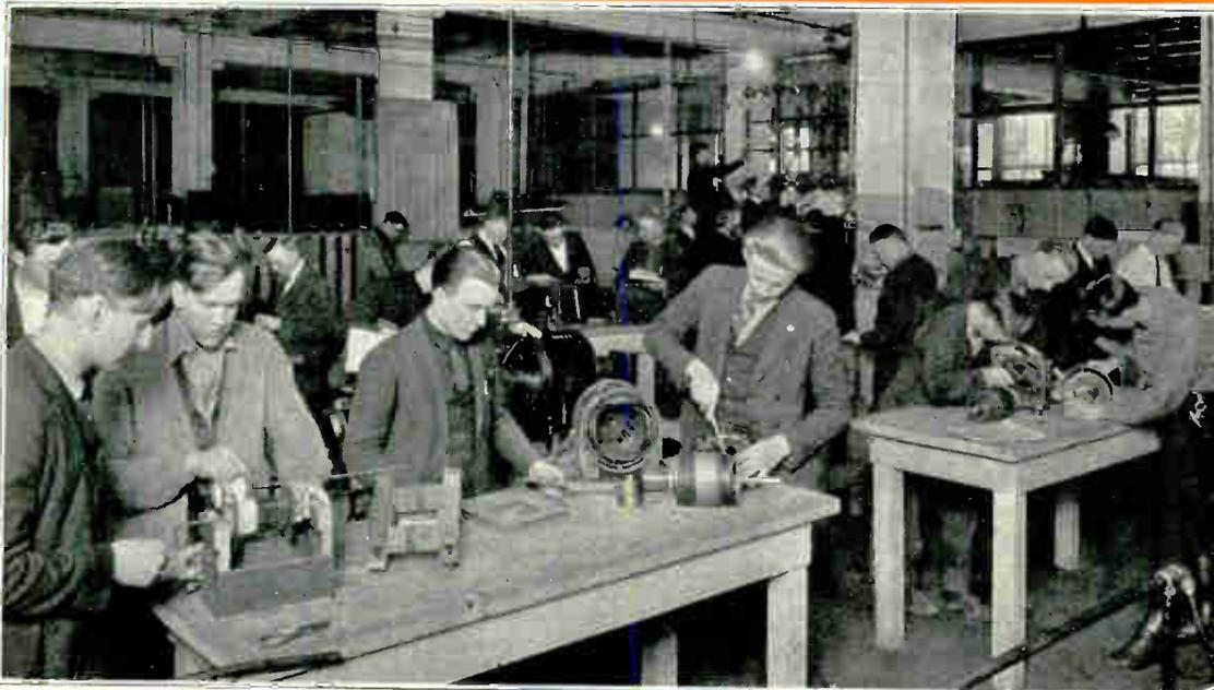
And these fellows are doing general trouble shooting and repair on A. C. motors, and building a complete test transformer for high voltage testing of insulation.
