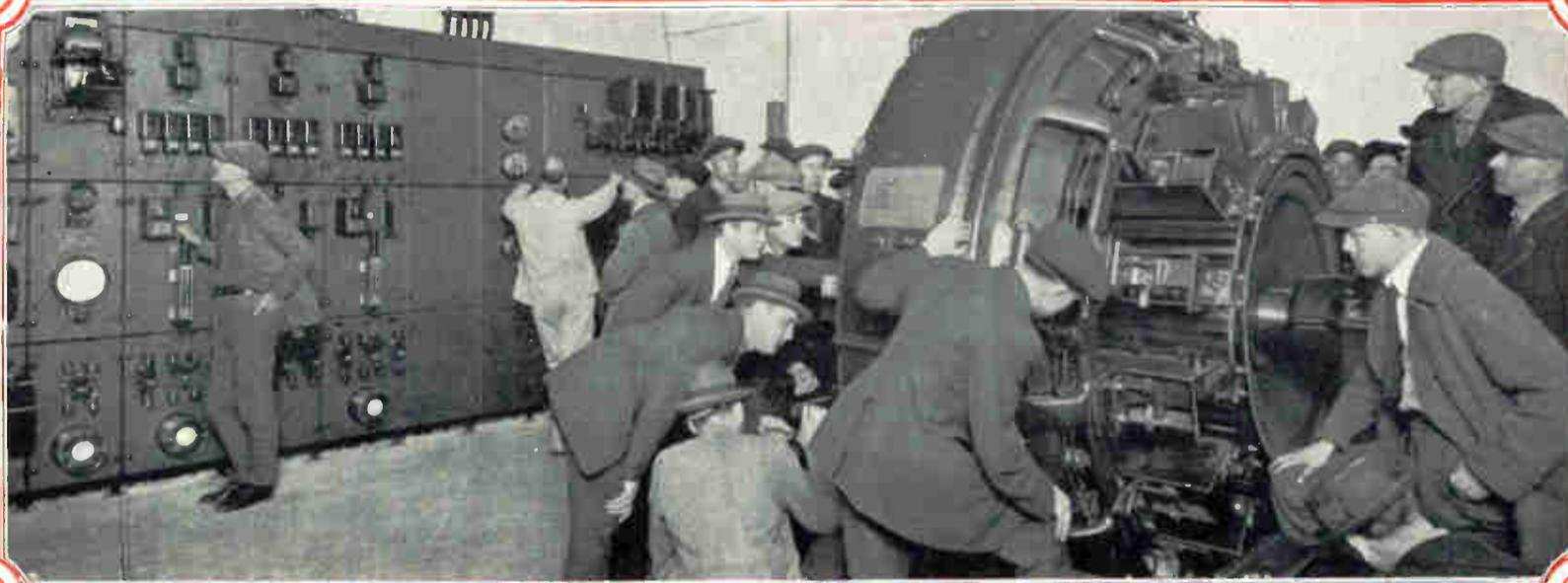
This is an automatic substation of the street railway systems, and the students are shown examining the 2000 K. W. converter, and switchboard. Trips to such plants as these are intensely interesting.
