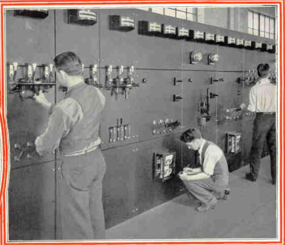
And these students are getting actual operating practice on a large A. C. switchboard. Here they are taught the operation and care of meters, circuit breakers and switches, and how to synchronize and operate alternators in parallel and equalize their load.
