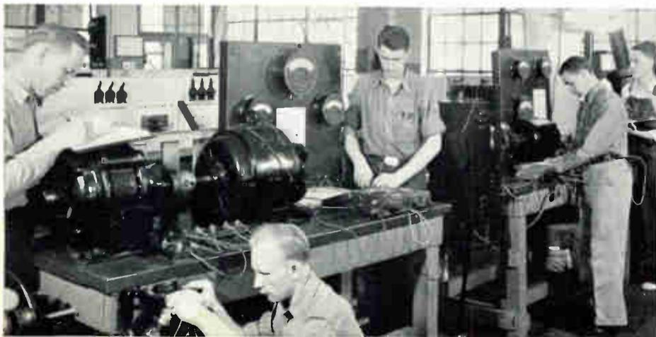
These students are testing the horsepower, efficiency, and power factor of induction motors, essential training for the practical maintenance man.
