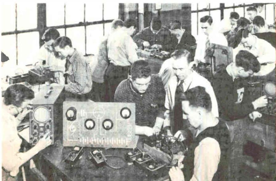
Here you see an Instructor giving students in our Industrial Electronics Department special instruction in checking the characteristics of high vacuum type tubes, using a specially constructed testing unit.
