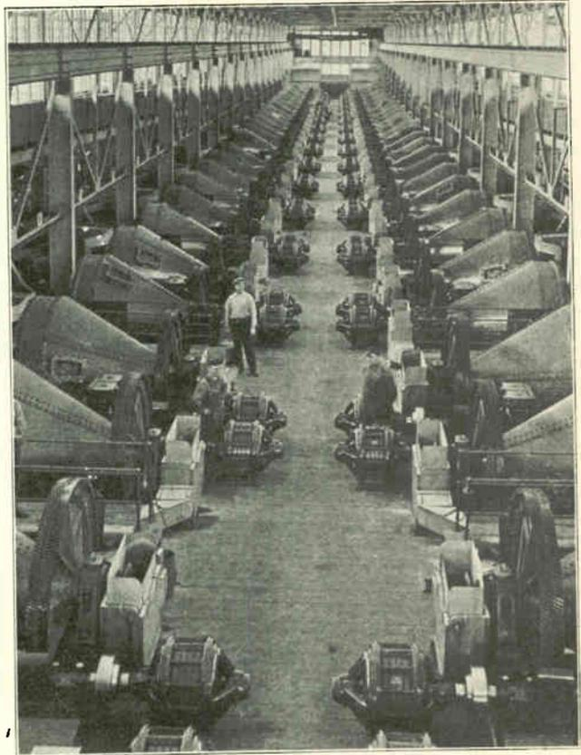
Fig. 475. This photo shows an installation of A. C. motors in a copper mill. Hundreds of thousands of motors in thousands of electrified factories and plants require the services of trained electrical maintenance men.
