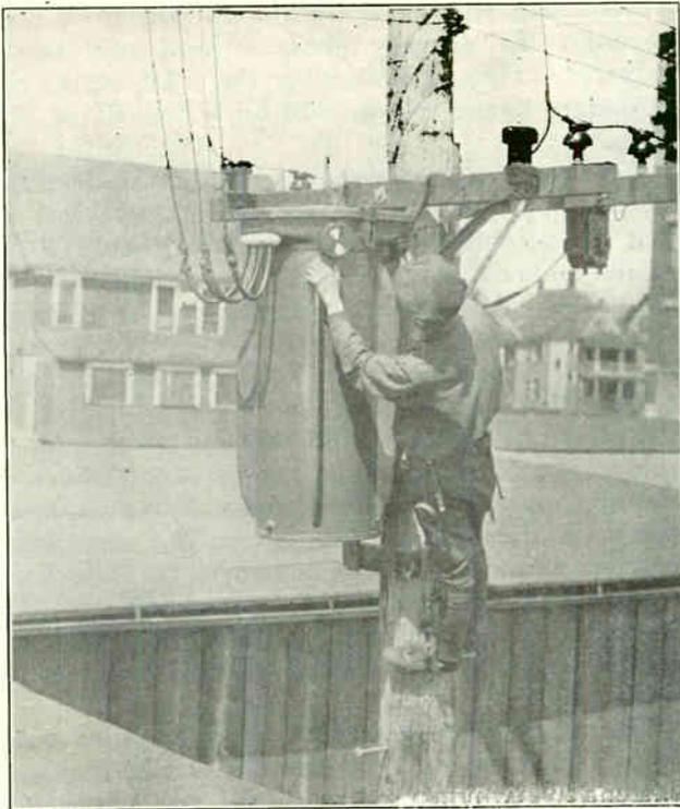
Fig. 124. This photo shows a pole type transformer and the method of making primary and secondary connections. Also note the thermotemperature indicator near the hand of the electrician.
