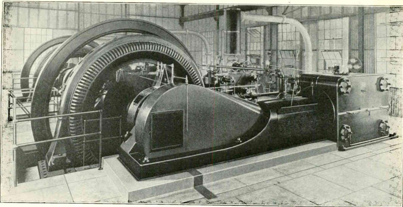
Fig. 83. This photo shows a view in a power plant equipped with horizontal type steam-engine-driven alternators. These alternators are made with large diameters because of the relatively low speed at which they are driven. (Photo Courtesy Allis Chalmers Mfg. Co.)
