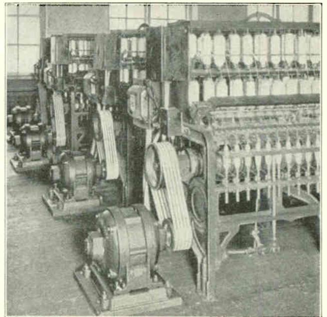
Fig. 154. This photo shows a group of machines in a textile mill, each of which is driven by an individual A. C. motor.
