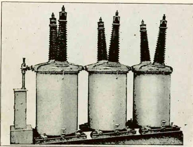
Fig. 427. Large outdoor oil switch for use in three-phase, 150,000-volt circuits. (Courtesy of Condit Electric Mfg. Co.)
