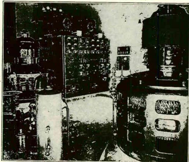
Fig. 321. Interior view of a small automatic hydro-electric generating station. The two generators can be seen in the foreground, and the switchboard in the background of this photo. (Courtesy Allis-Chalmers Mfg. Co.)
