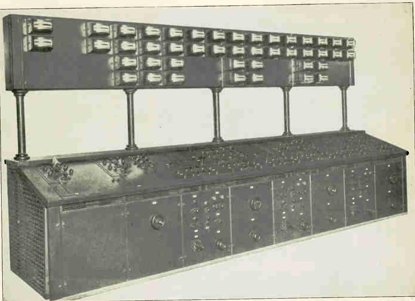
Fig. 417. Modern bench-type switchboard for remote control of generators and oil switches in a large central station. Note the arrangement of the meters and the push-pull switches which control the solenoid operated and motor-operated oil switches and devices throughout the plant. (Courtesy of G. E. Company.)
