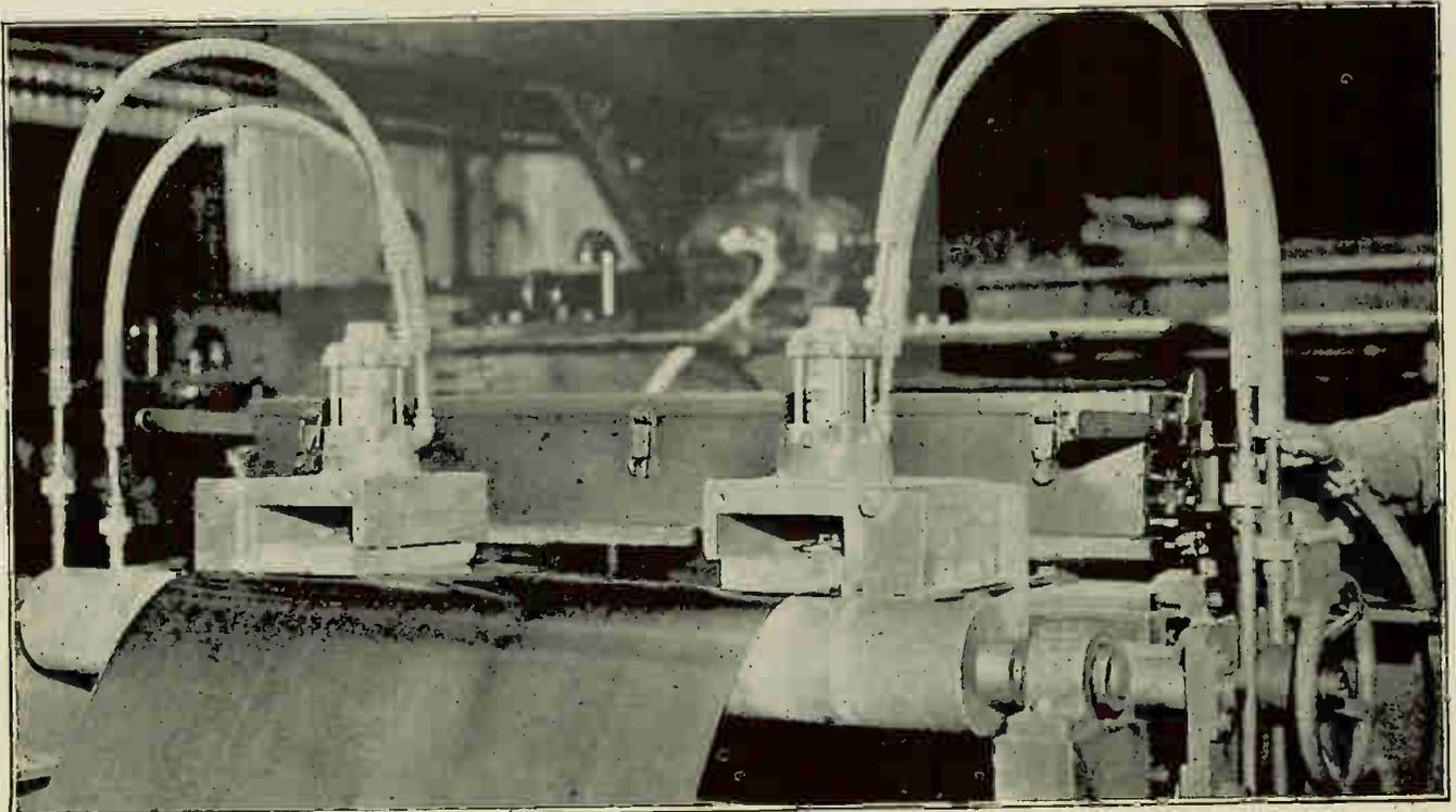
Electro-lytic cleaning and sharing line for 10 plate. View showing scanning head for pin hole detector with manually operated side guides, each maintains strip at proper pass line. "P" means air operated pressure blocks. Scanning head operated by compressed air. G. E. pine hole detector and marking device.
