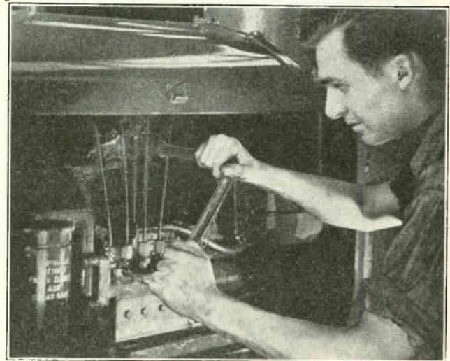
Fig. 77. This photo shows an operator attaching the hand crank to shift the valves for starting an International Harvester Diesel on gasoline fuel.
