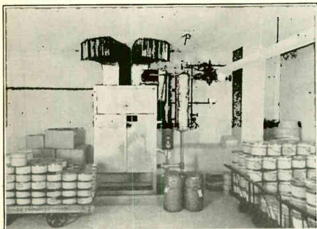
Fig. 173. Commercial unit type air conditioner for storage rooms, etc. Courtesy Carrier Corp.
