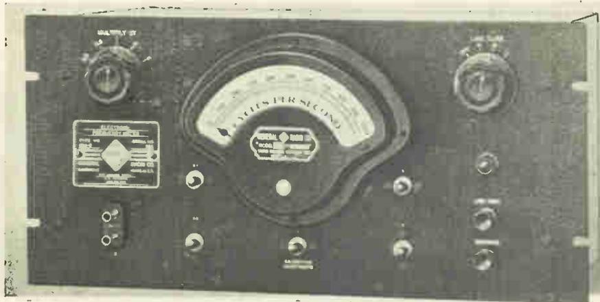
Precision panel-mounted electronic frequency meter.
