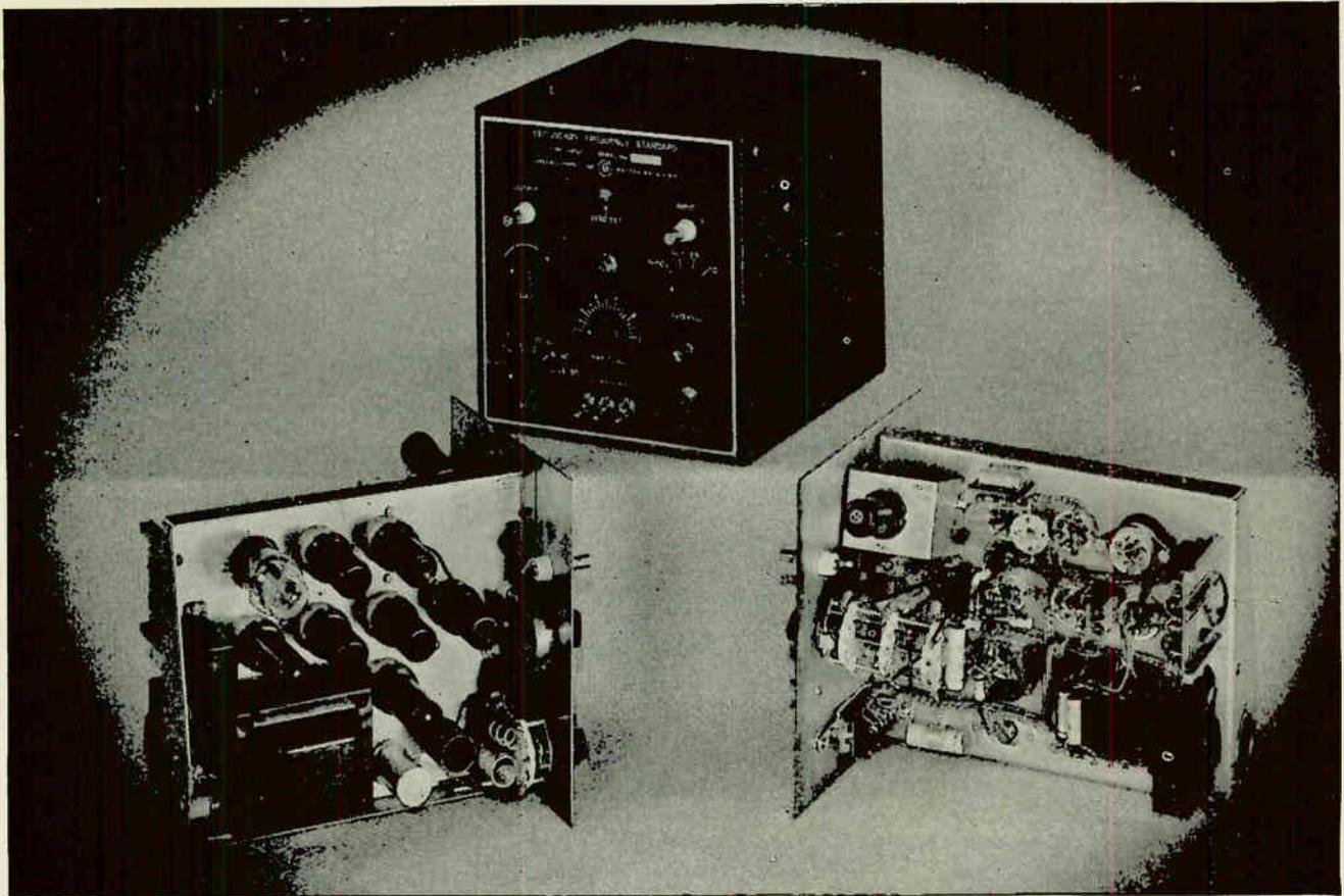
Crystal-controlled secondary frequency standard for checking transmitter wave length.
