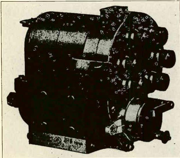
Fig. 48. Photograph of a high tension magneto used for ignition purposes on trucks, busses, tractors, etc. Courtesy Bosch Magneto Corporation.
