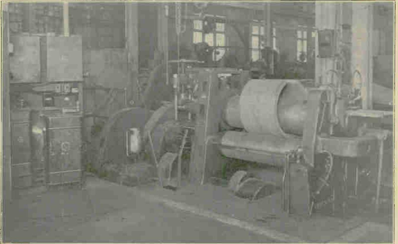
Bending roll equipped with G. E. Electro Magnetic strain gage equipment. Instruments over controller show rated load during rolling operations. Alarm given when machine load exceeds rated capacity.
