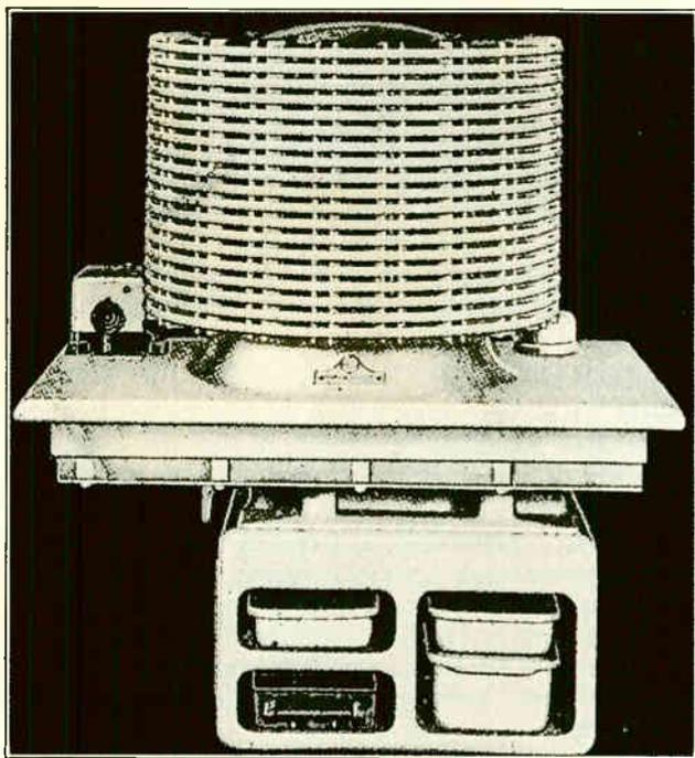
Fig. 78. Above is shown one type of General Electric refrigerating unit which can be quickly removed from the top of the cabinet for replacement by another unit in case of any defect or service requirement. Note the condenser coil located around the hermetically sealed motor and compressor unit. Courtesy General Electric Company.
