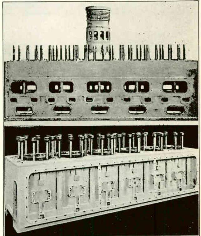
Fig. 136. In the top view is shown the upper section of a Diesel engine frame or cylinder block with one of the cylinder liners removed. In the bottom view is shown a six cylinder engine block with the liners all in place.
