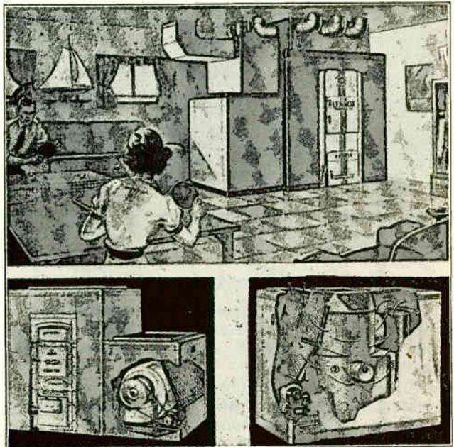
Fig. 142. Upper view shows a combined furnace and air cooling and cleaning unit, or summer and winter air conditioner installed in the basement of a home. The lower views show cut-away views on these units. Courtesy Lennox Furnace Co.
