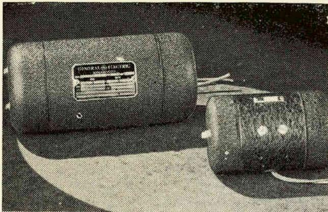
Motor generators must be filtered to by-pass interference to radio receivers.
