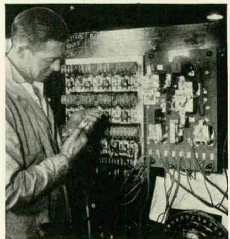
One common source of interference is loose or dirty contacts in fuse boxes or other electrical units.
