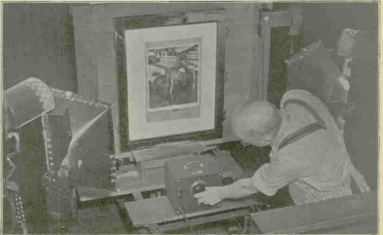
A Totalux being used to integrate light intensity with time, in reference to exposure in photography.
