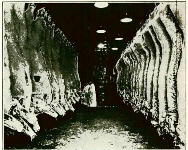
Fig. 20. Photograph of one section of a large meat chilling and storage room which is kept at very low temperature by means of mechanical refrigeration. Courtesy Carrier Corporation.
