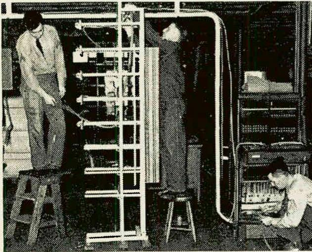
This type of installation is seldom the cause of man-made interference. Everything is tied down and careful soldering prevents sparking.
