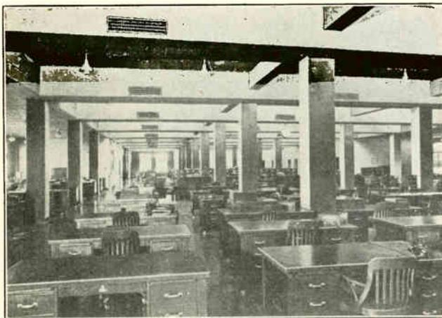
Fig. 148. Photo of the inside of a modern air-conditioned general office. Note the duct outlets along the ceiling beams. Much better efficiency and health can be maintained in such air-conditioned offices. Courtesy Jewell Tea Co.
