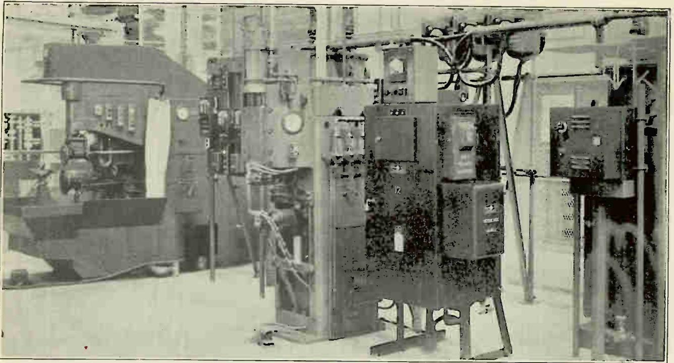
Resistance Welding Area. General front view showing 200 KVA seam Welding Machine and 75 KVA Welding Press with associated equipment, including 2300 to 460 volts distribution transformer.
