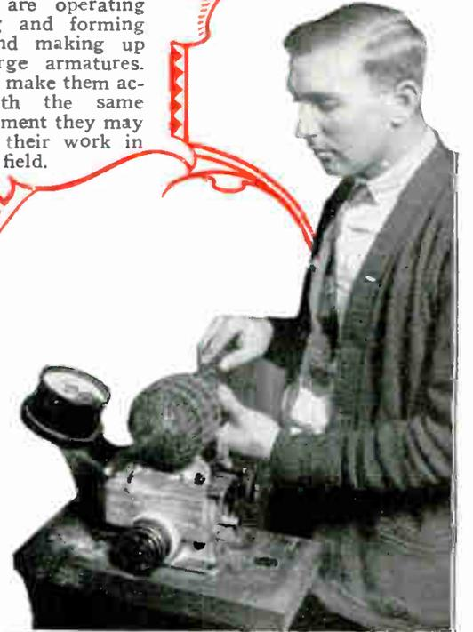
This Student is testing an armature on the growler, a machine for quickly locating trouble and faults in windings. This kind of instruction helps our graduates to get right at the cause of armature troubles without waste of time.
