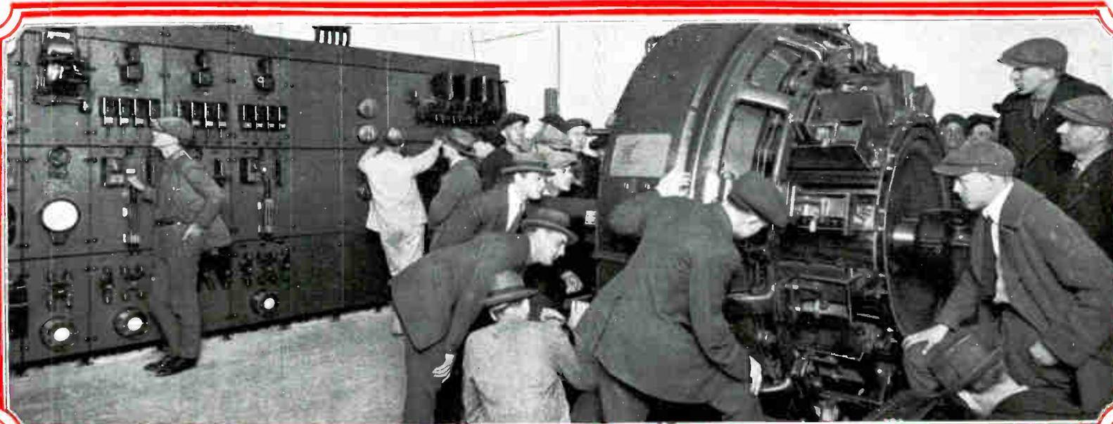
This is an automatic substation of the street railway systems, and the students are shown examining the 2000 K. W. converter, and switchboard. Trips to such plants as these are intensely interesting.
