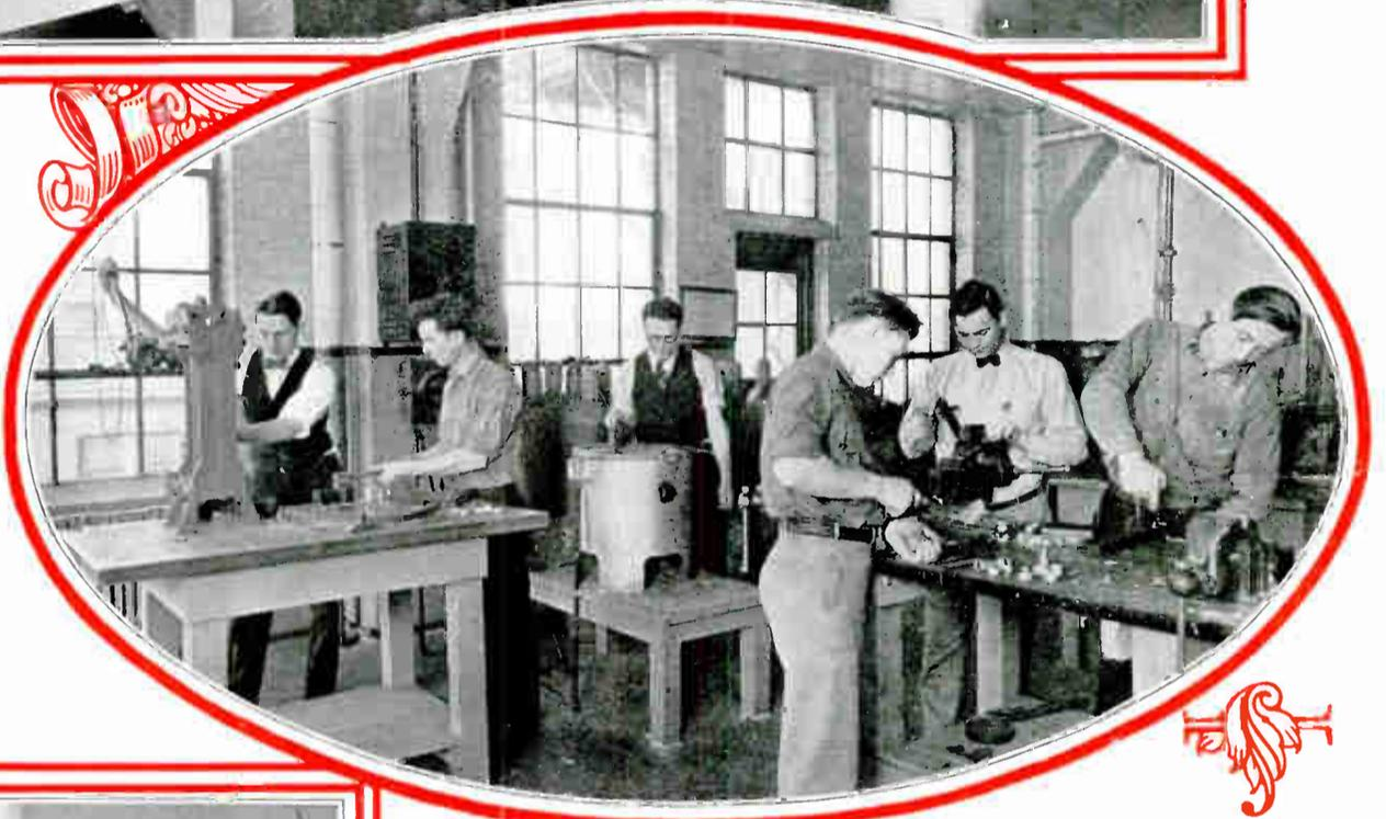
And these students are melting lead in an electric melting pot, and moulding lead posts and straps for the batteries they are building. This work gives them excellent practice with tools, and modern equipment.
