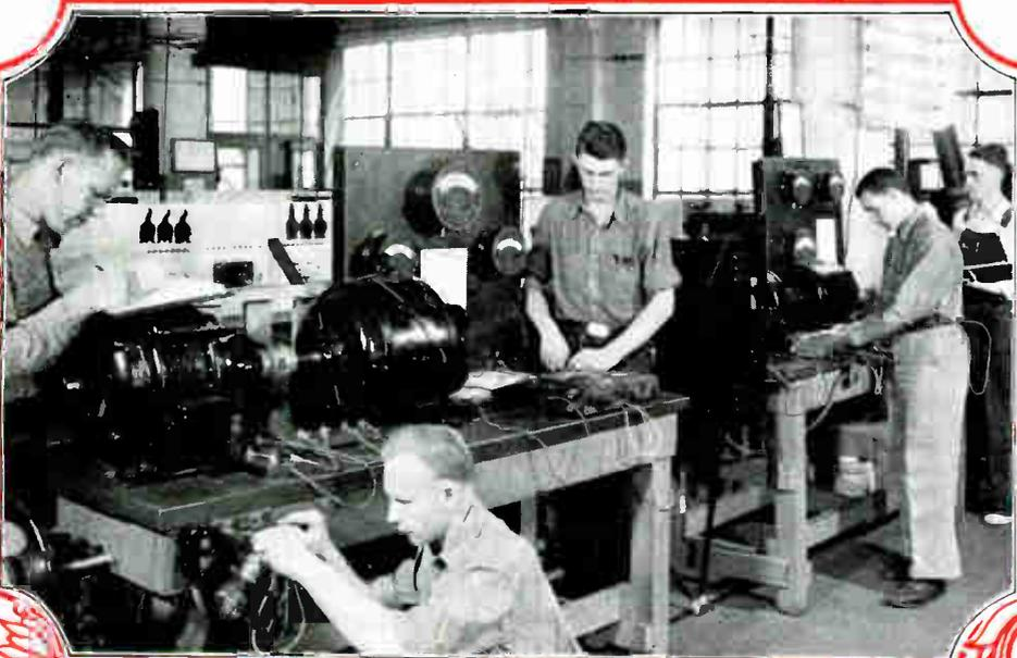
These students are testing the horsepower, efficiency, and power factor of induction motors, all very valuable things for the practical maintenance man to know.
