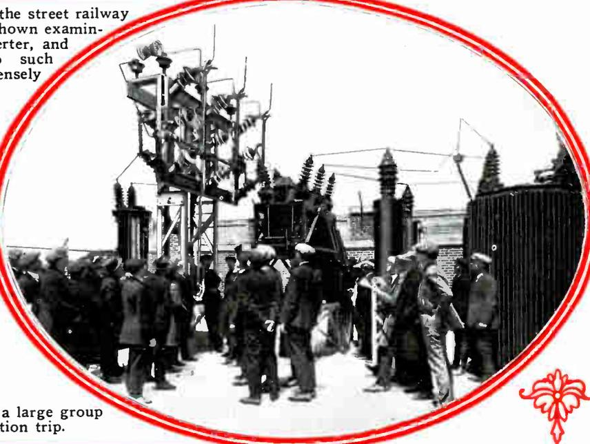
The oval picture above is of an outdoor substation and these students are examining the oil switches, lighting arresters and transformers, with instructors along to explain everything.
