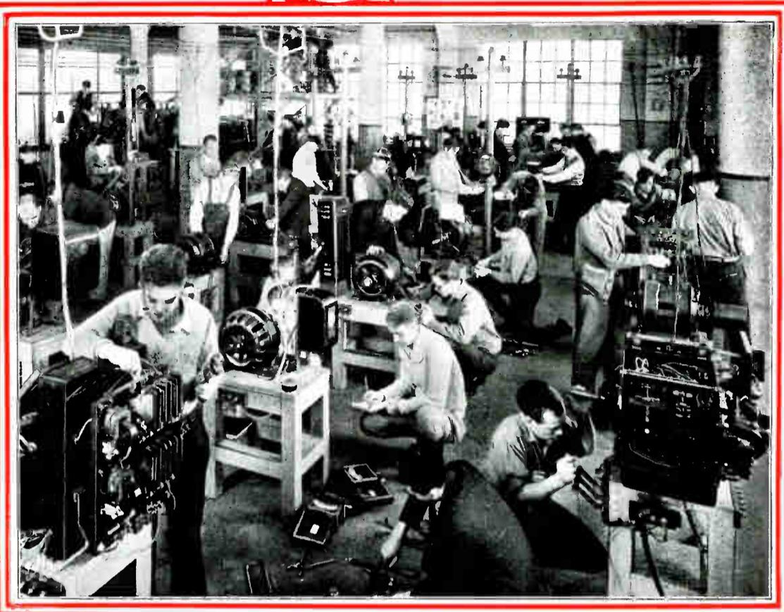
Another view of a section of our A. C. department showing students working on a wide variety of A. C. motors and control equipment. You learn how to inspect, connect up, test and repair many types of A. C. machines. This practical training in modern maintenance work helps to make Coyne Graduates more valuable to their employers.
