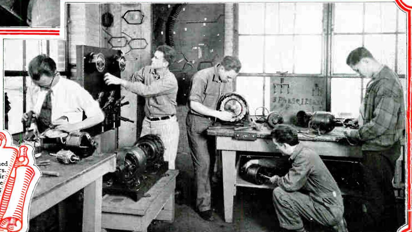
These students are testing finished winding of armatures and stators. This is the way they find their mistakes and are taught to make their windings correct. Testing armatures and stators and locating faults in the windings, is very valuable to any maintenance man.
