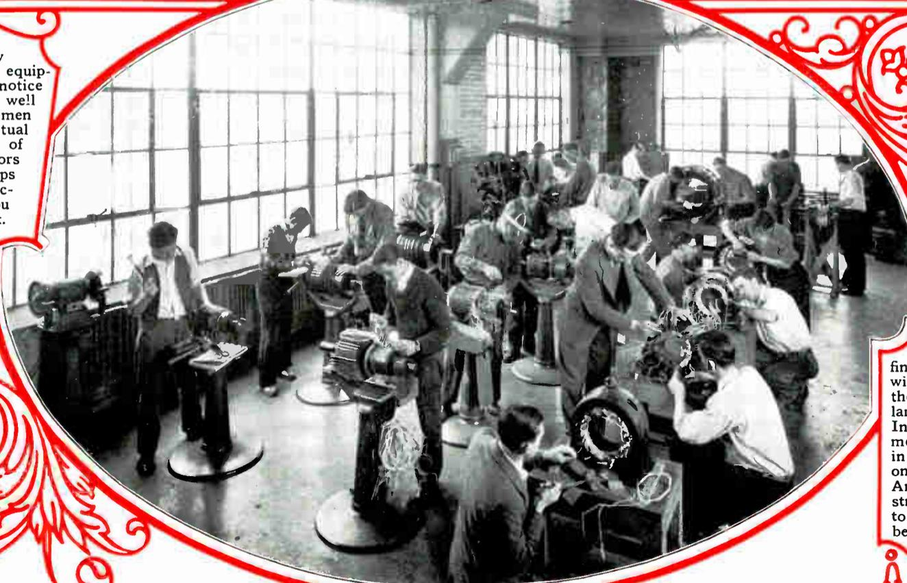
These students have finished their first small windings and here you can see them winding and testing large armatures and stators. In the background you see men truing up a commutator in a lathe and others working on a 100 H. P. A. C. stator. And in the foreground, instructor shows a student how to test his finished winding, before connecting up the leads.
