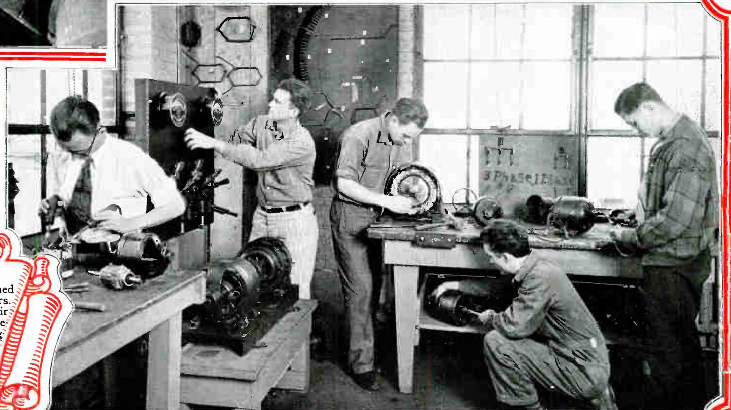
These students are testing finished winding of armatures and stators. This is the way they find their mistakes and are taught to make their windings correct. Testing armatures and stators and locating faults in the windings, is very valuable to any maintenance man.
