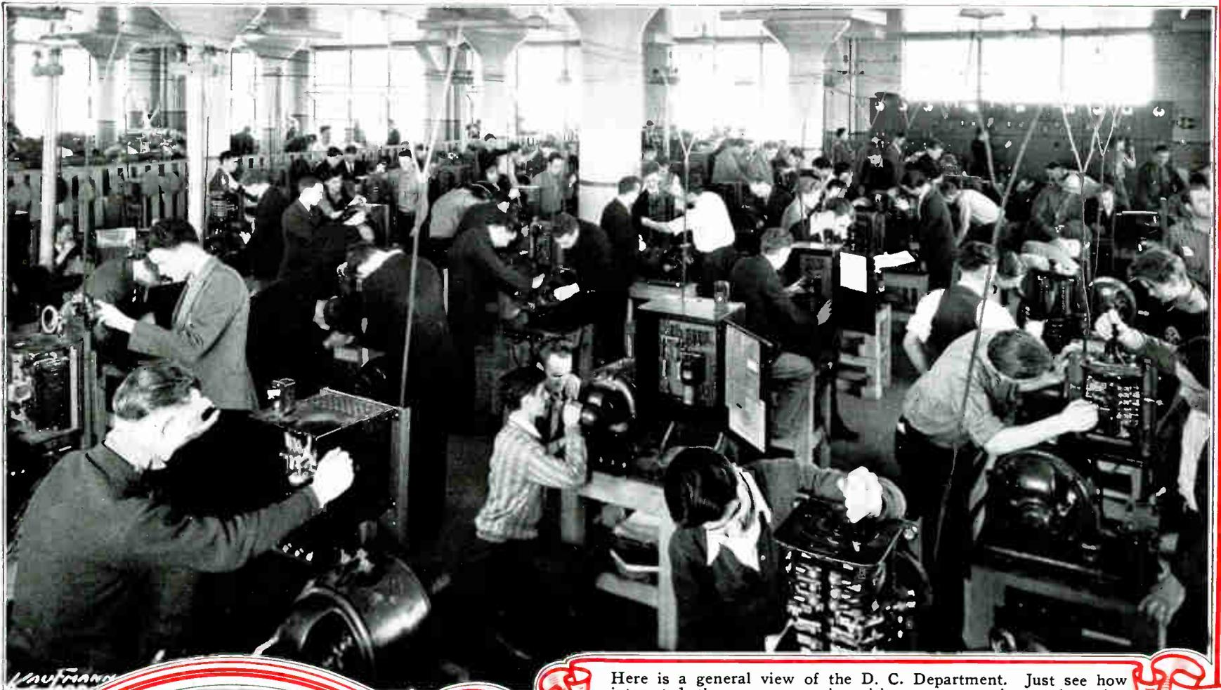
Here is a general view of the D. C. Department. Just see how interested these men are in wiring up, operating and testing D. C. motors and controllers of all common types. These machines are supplied with power from the generators right in this department.
