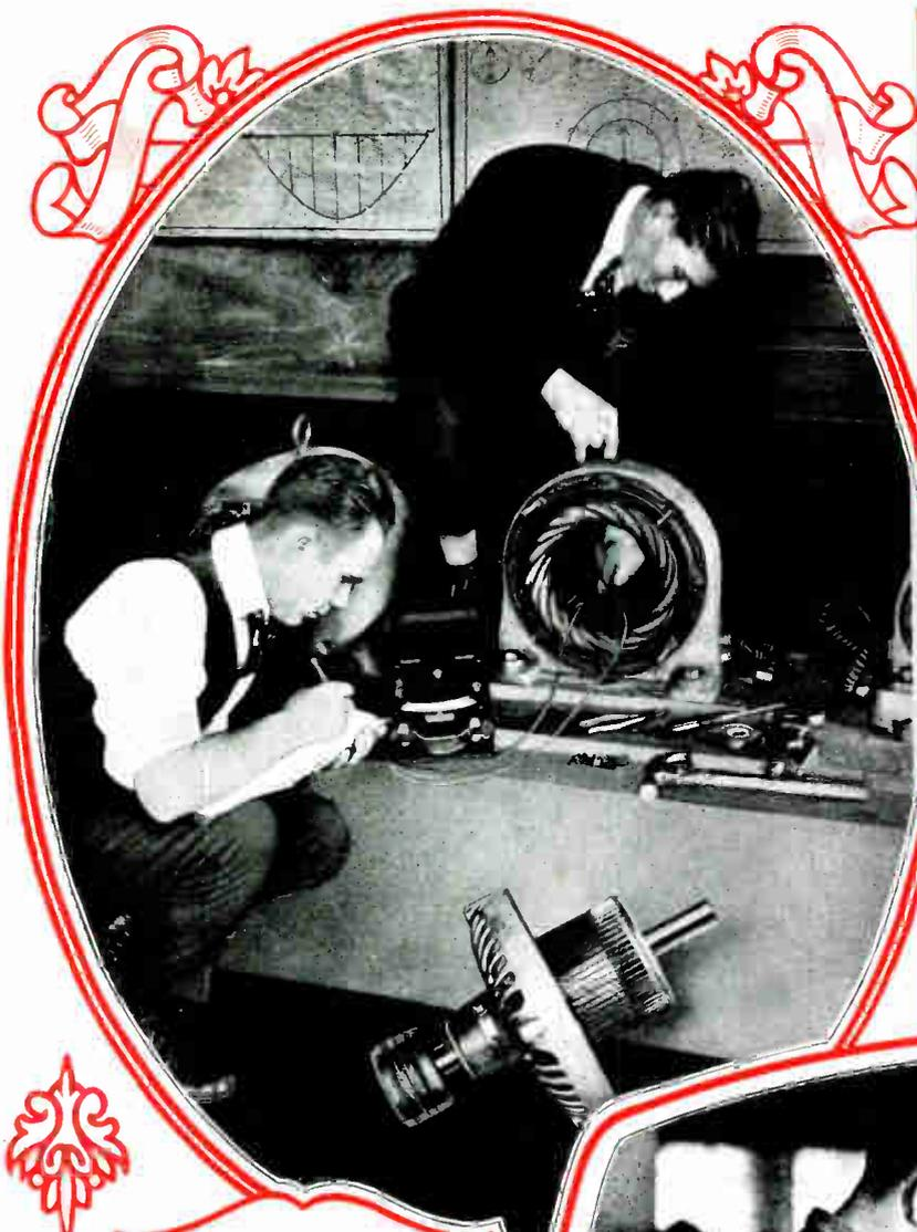
Real practical work overhauling and repairing an A. C. induction motor. When you understand the working parts of such equipment you have confidence in your knowledge of this work.
