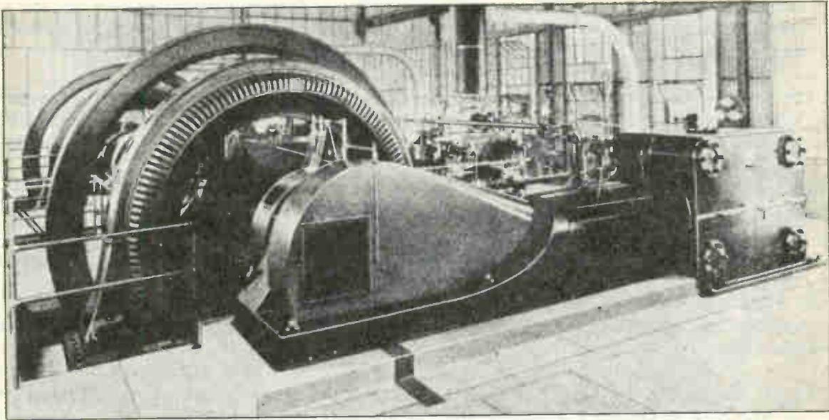
Fig. 5. This photo shows a view in a power plant equipped with horizontal type steam-engine-driven alternators. These alternators are made with large diameters because of the relatively low speed at which they are driven.
