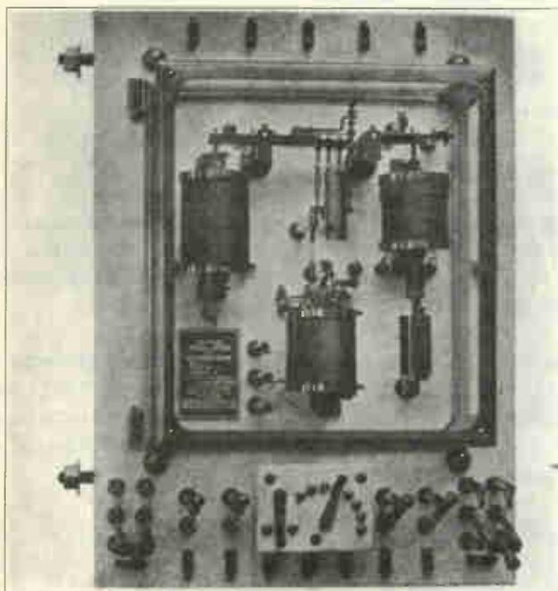
Fig. 15. This photo shows an automatic voltage regulator of a type similar to the one for which the wiring was shown in Fig. 10, and shows the arrangement of the solenoids and relays on the panel.
