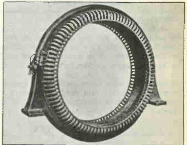
Fig. 2 Above is shown the stator of a large synchronous motor. You will note that the stator, frame, core, and windings are the same as those used for alternators.
