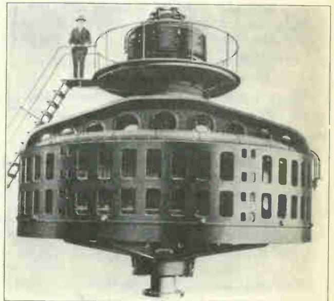
Fig. 4. Large vertical type alternator for water-wheel drive. The stator core and windings of this machine lay in a horizontal position just inside the lower frame work, and the field poles revolve on the vertical shaft within the stator.
