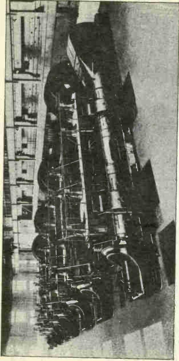
Fig. 4 Privately owned power plant producing alternating current for use in steel mill operations. These alternators are driven by gas engines which burn waste gases as a fuel.
