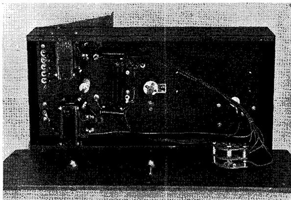
*Fig. 1036* — The individual filament transformers are small enough to be mounted inside the chassis. Grid leaks and meter-shunting resistances are mounted between fibre lug strips. The shaft of the grid tank condenser is fitted with an insulating coupling. Meter-switch leads are cabled and connection to the switch made just before the panel is fastened to the 8 in.-by-17 in.-by-3 in. chassis.
