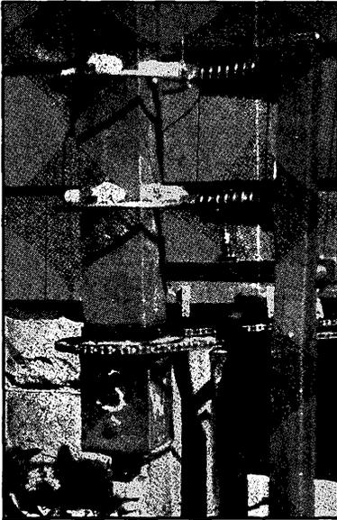
Fig. 2507 — One form of rotating mechanism. A bicycle sprocket and chain turn the pole which supports the beam antenna. Feeder connections from the antenna are brought to the metal rings, which slide against spring contacts mounted on the large stand-offs on the short pole.
