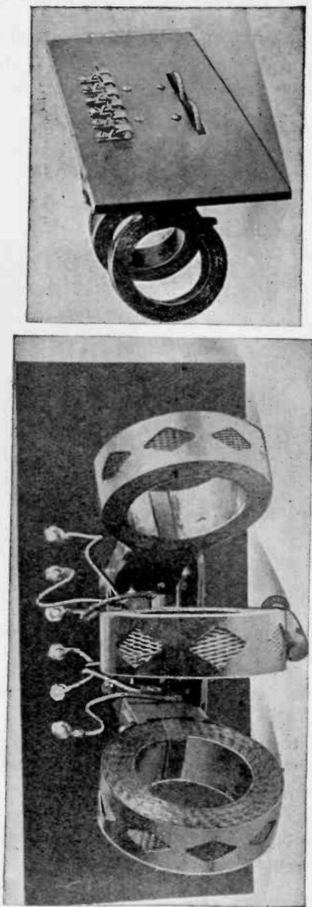
Fig. 36.—A loose coupler for damped or undamped waves. Coils of this size are made with inductance values up to 175 millihenries.
