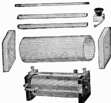
Fig. 8.—Details of the tuning coil
