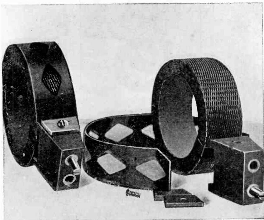
Fig. 35.—Showing how the honeycomb coils are made up on plugs for mounting.
