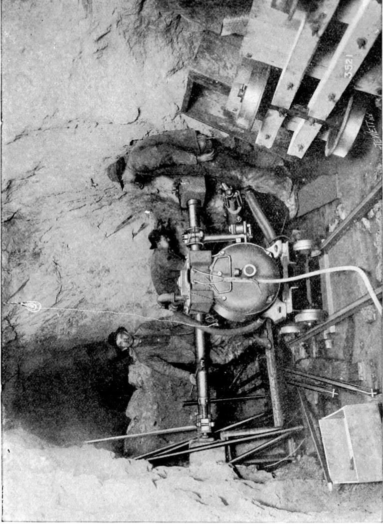
AN ELECTRIC-COMPRESSED-AIR DRILL IN THE "SEVEN MILE TUNNEL," DUMONT, COLORADO
