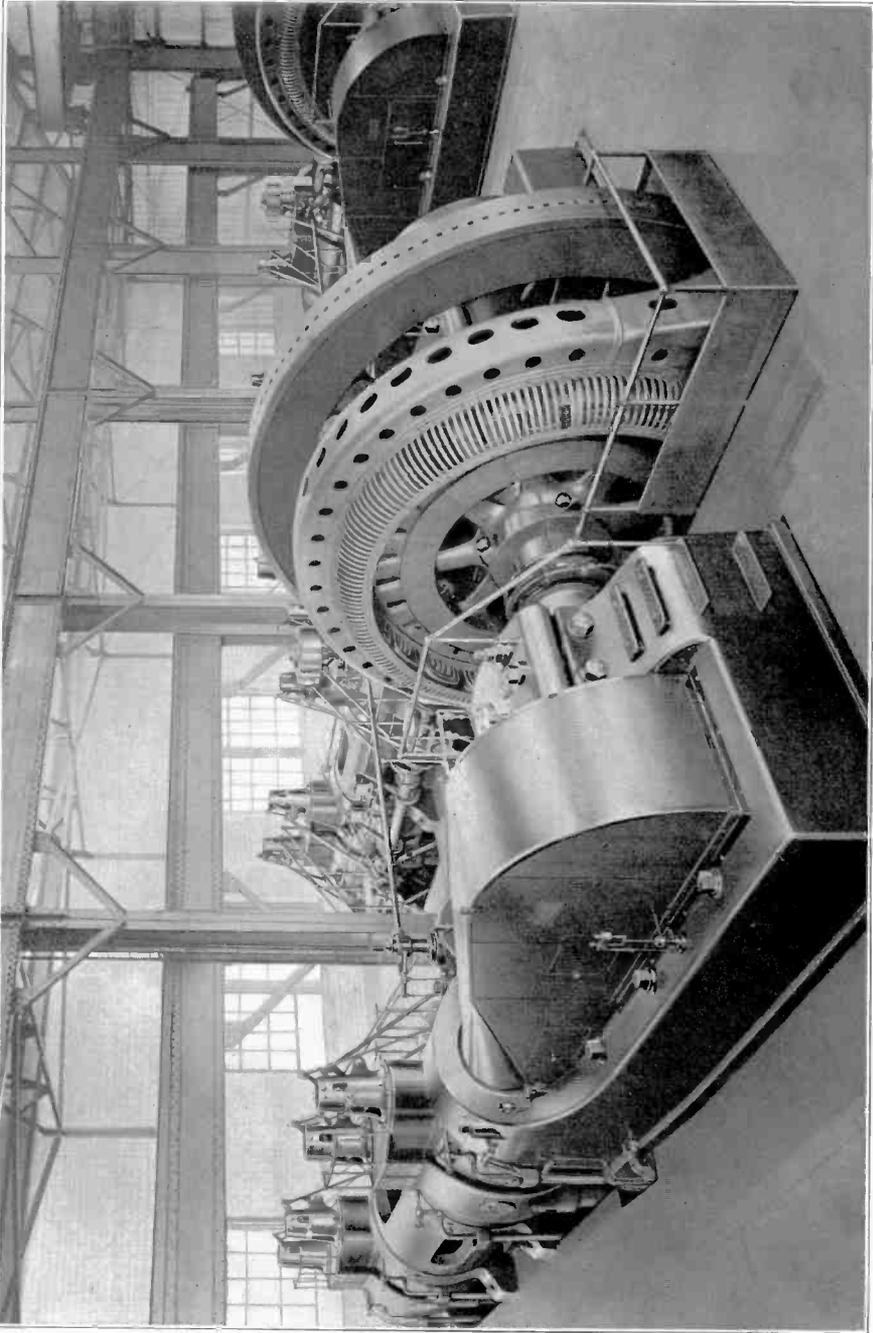
ONE OF FOUR 1500-H. P., FOUR-CYCLE, DOUBLE-ACTING, GAS ENGINES, EACH DRIVING A 1000-Kw. ALTERNATING-CURRENT GENERATOR
