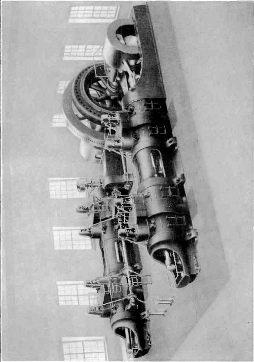
**FOUR-CYCLE, DOUBLE-ACTING, TWIN-TANDEM GAS ENGINE DIRECT-COUPLED TO ALTERNATING-CURRENT GENERATOR**
