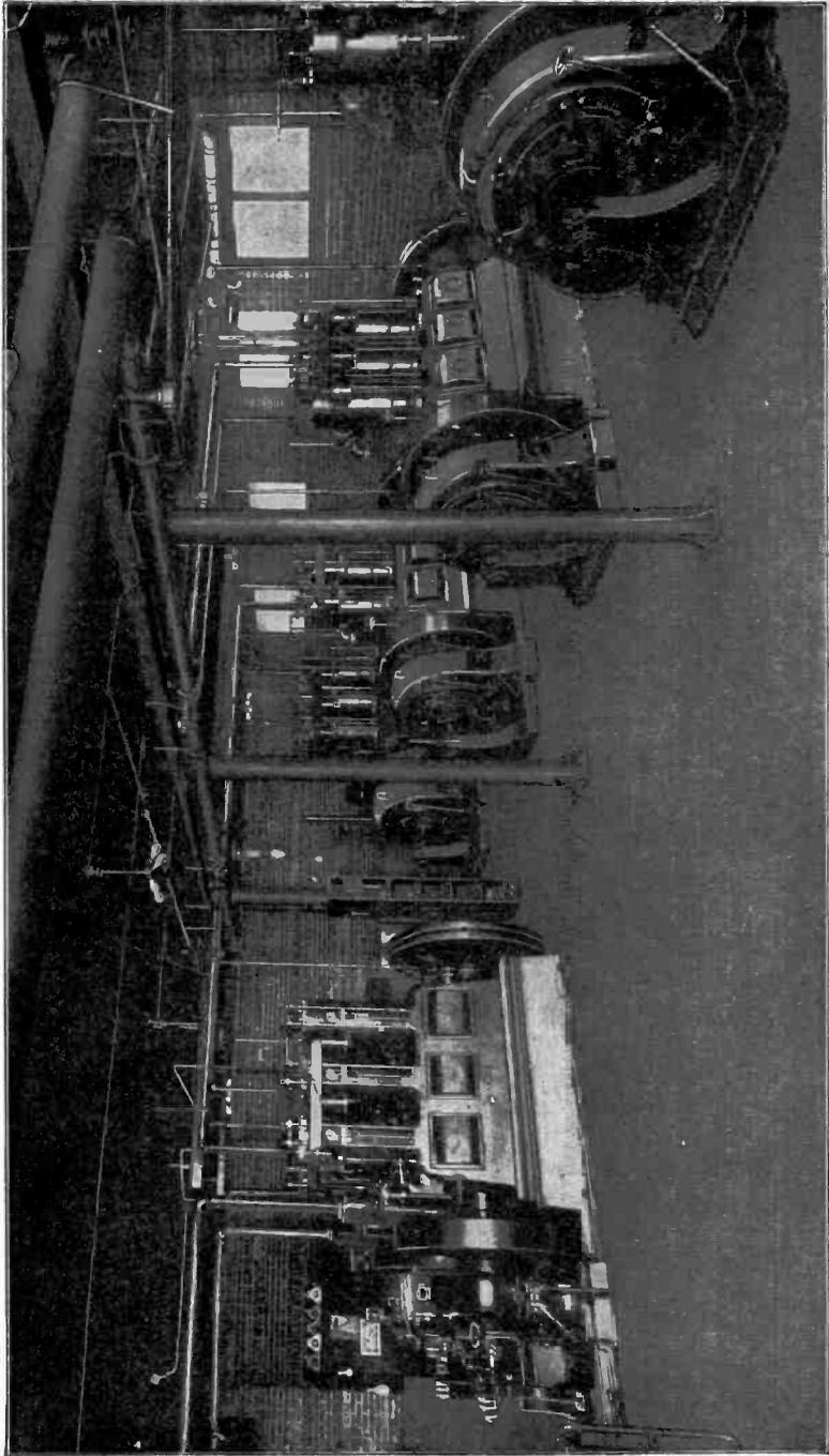
**WALRATH GAS ENGINES DIRECT CONNECTED TO GENERATORS**
