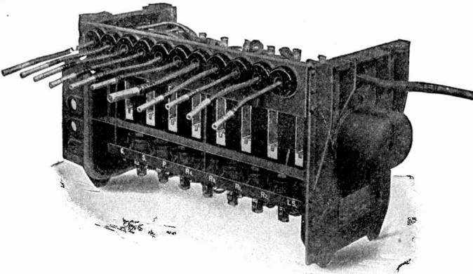
Fig. 71. Group of Unit Switches, Westinghouse System
