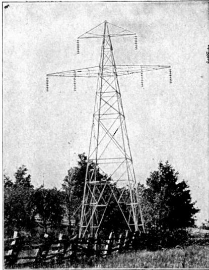
Fig. 178. Modern High-Tension Tower with Suspension Insulators
