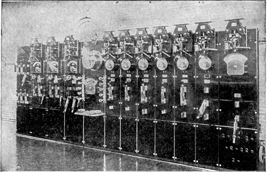
Fig. 151. Simple Railway Switchboard Panel
