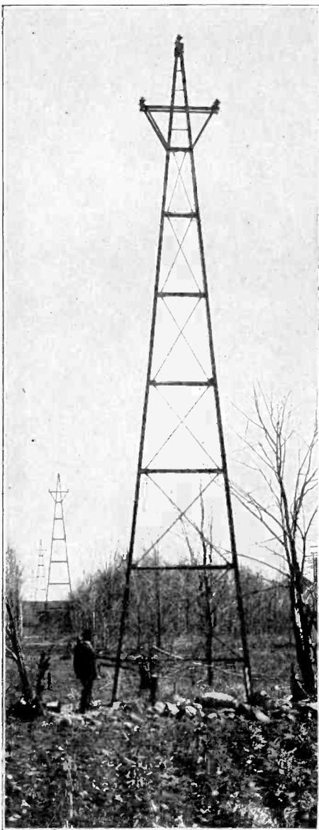
Fig. 174. Steel Tower with only Side Bracing
