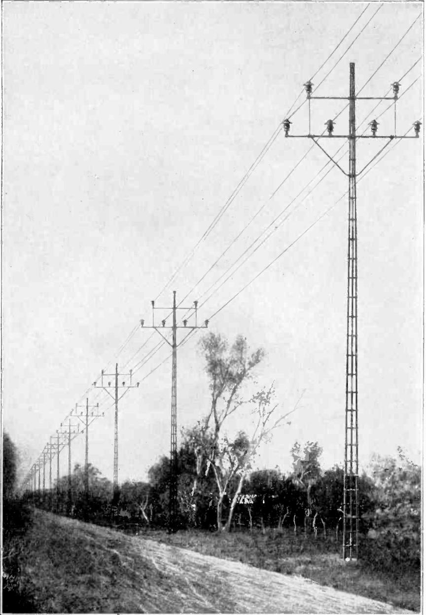
Fig. 173. Steel Pole Construction for High-Tension Circuit
