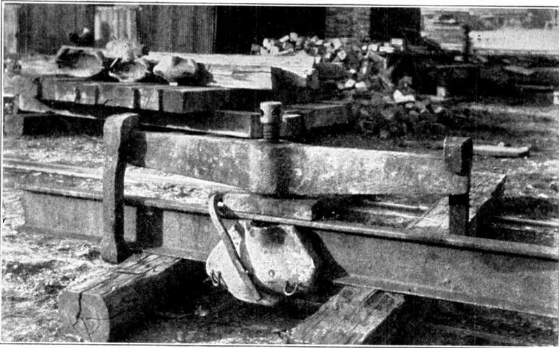
Fig. 229. Apparatus Set for a Cast-Welded Joint
