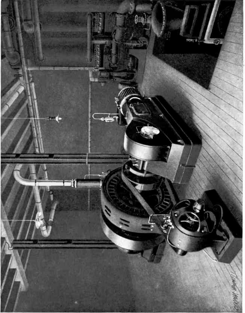
HORIZONTAL CROSS-COMPOUND SINGLE-VALVE ENGINE, DIRECT-CONNECTED TO GENERATOR
