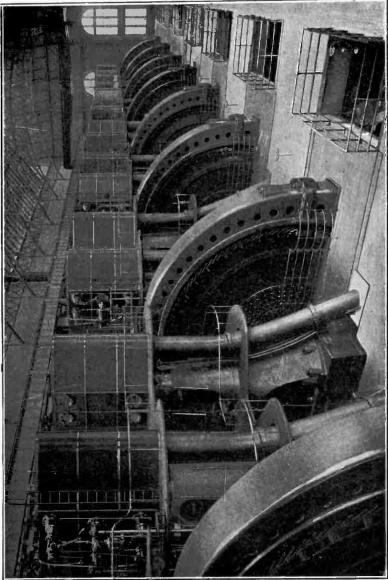
**EIGHT 5,000-K. W. GENERATORS, INSTALLED AT THE MANHATTAN STATION, NEW YORK CITY**
