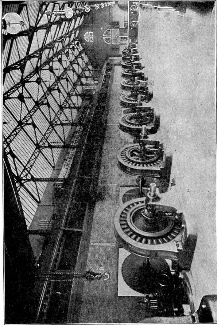
Fig. 55. Arrangement of Units in a Hydraulic Plant
