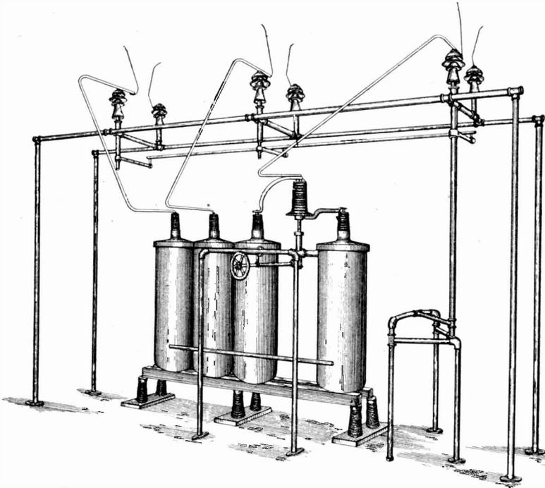
Fig. 37. Installation of Aluminum Lightning Arrester for 35,000 Volts
