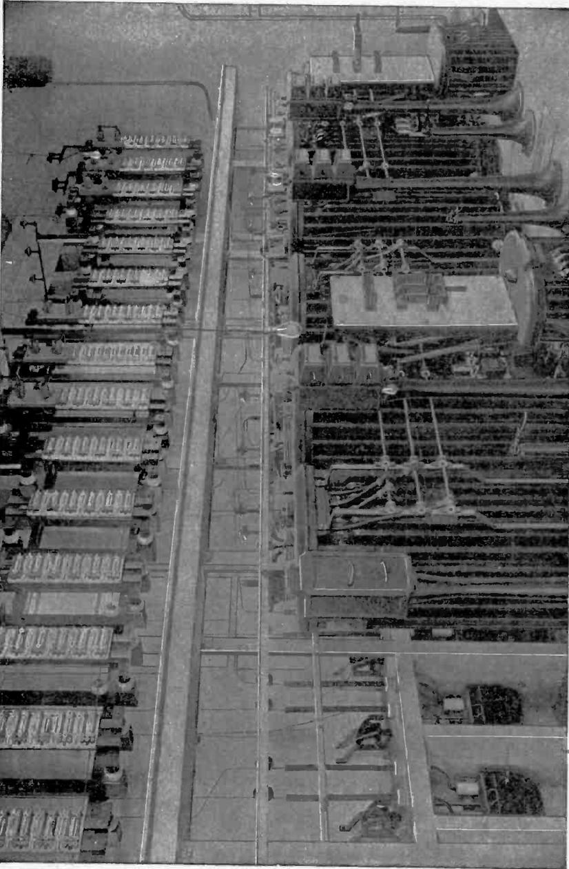
Fig. 35. Typical Installation of Lightning Arresters
