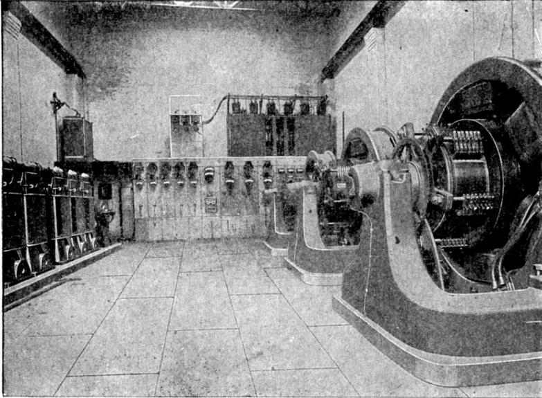
Fig. 56. A Good Arrangement of Apparatus for Substation
