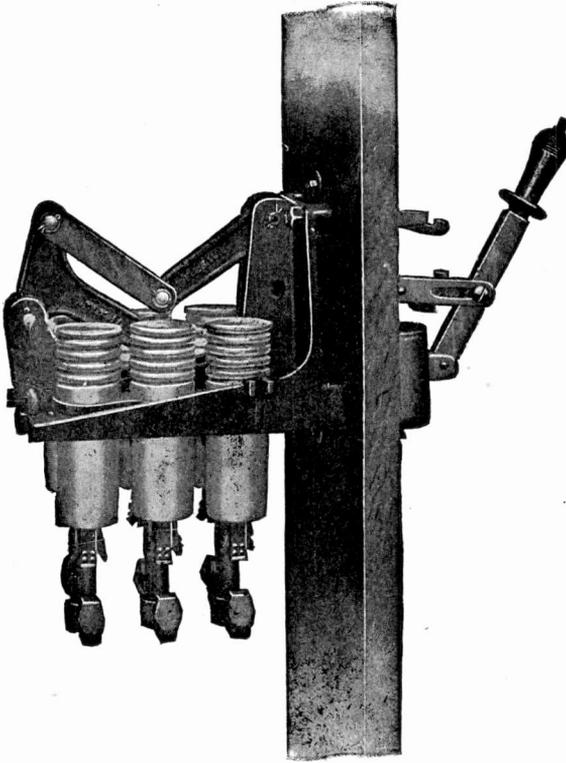
Fig. 26. Three-Phase Oil Switch with Oil Container Removed
