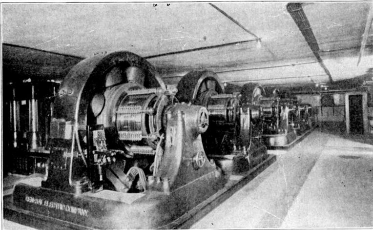
Fig. 21. Rotary Converters in Basement of Office Building.
