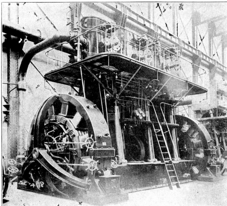
Fig. 8. 1200 H.P. Southwark Engine and 400 K.W. Generator.
