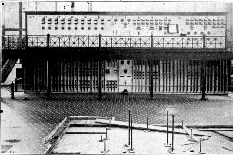
Fig. 18. Switchboard of 4-Wire 3-Phase Distribution System.
