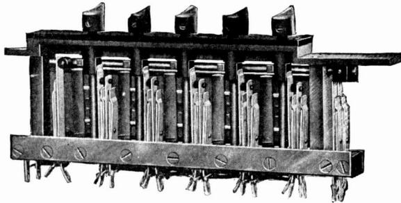
Fig 215. Western Electric Trunk Ringing Key
