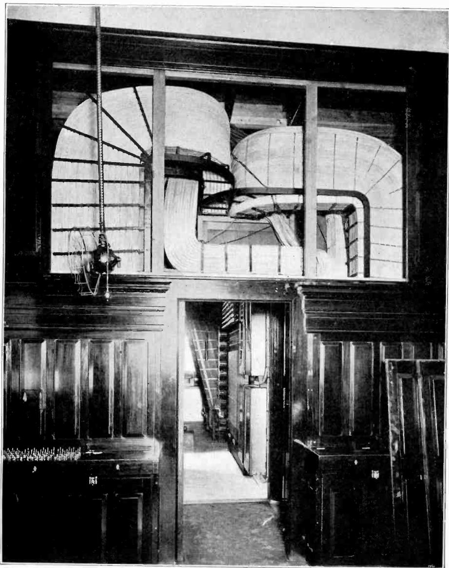
**CABLE TURNING SECTIONS, BETWEEN A AND B BOARDS**
