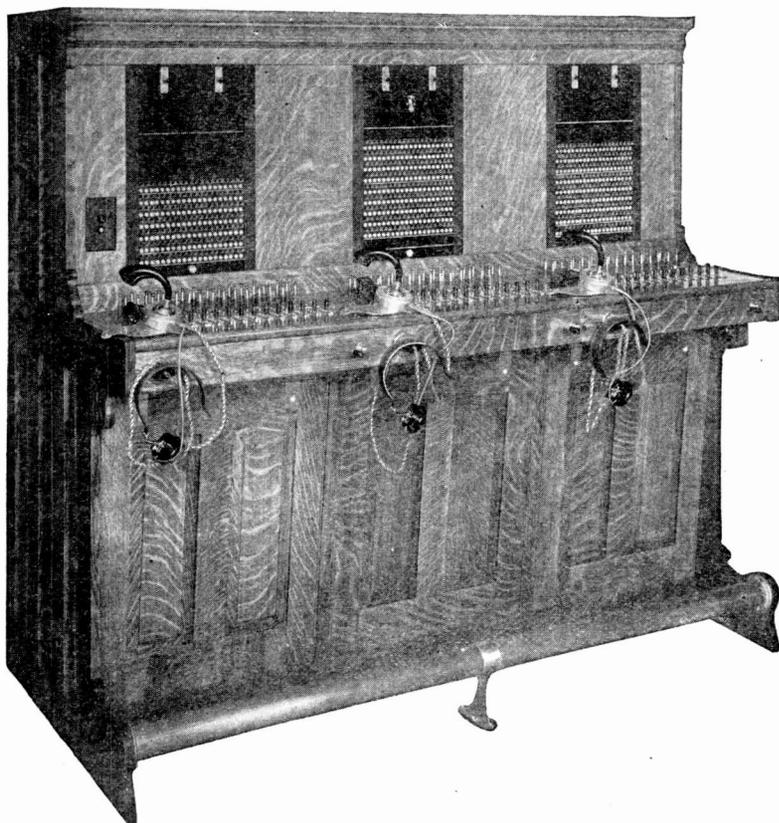
Fig. 177. Three-Position Lamp Board
