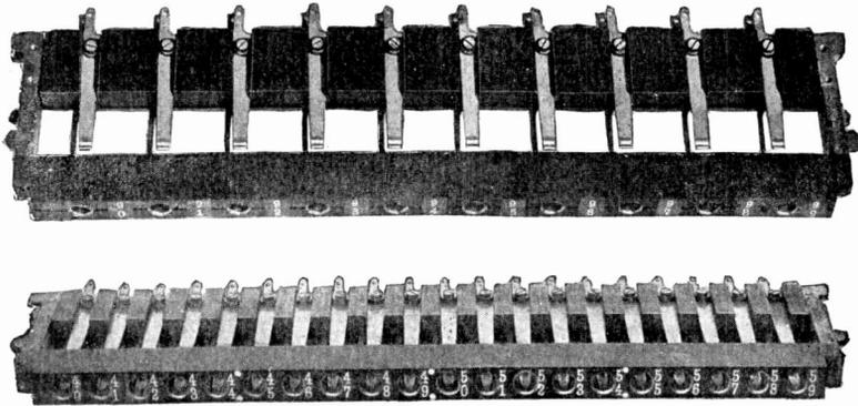
Fig. 202. Answering and Multiple Jacks for Kellogg Two-Wire Board
