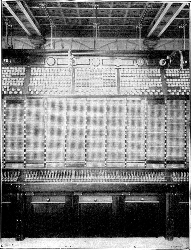
Fig. 181. Face of Magneto Multiple Switchboard
