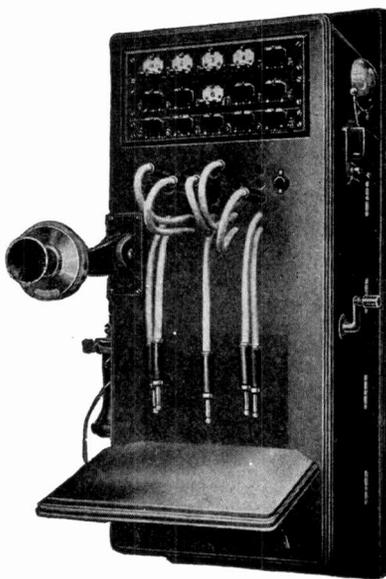
Fig. 141. Combined Telephone and Switchboard
