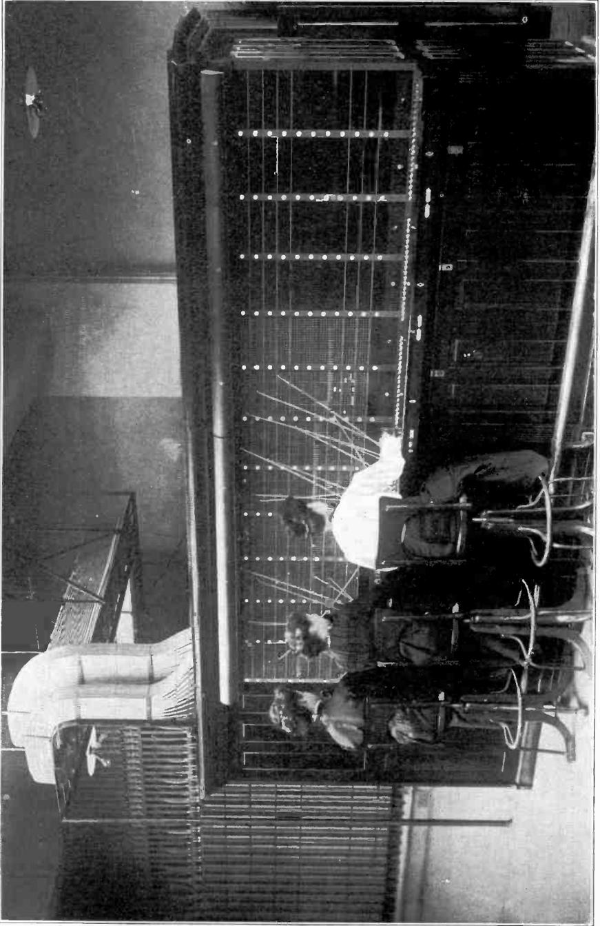
**A MULTIPLE MANUAL SWITCHING BOARD FOR TOLL CONNECTIONS IN AN AUTOMATIC SYSTEM**
