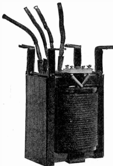
Fig. 242. Assembled "Remek" Core and Coils
