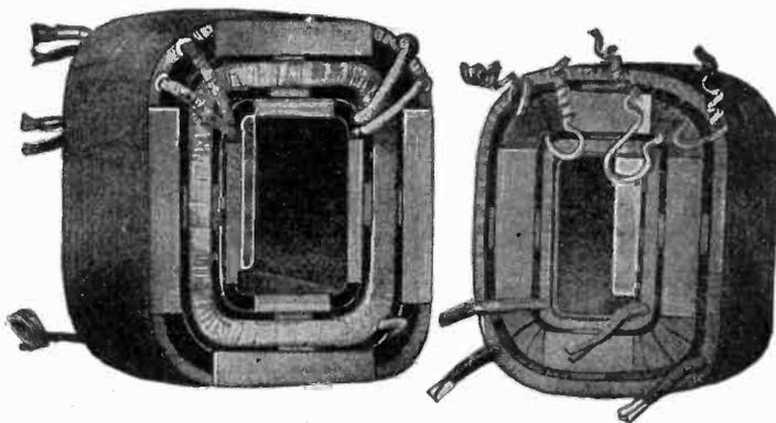
Fig. 247. Assembled Coils for Westinghouse Transformer
