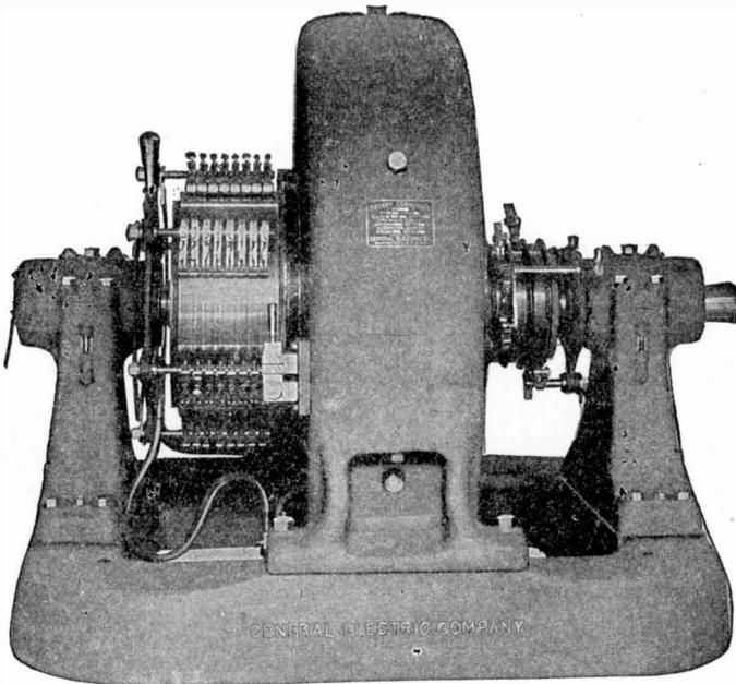
Fig. 299. General Electric 300-Kilowatt Three-phase Rotary Converter
