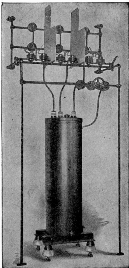
Fig. 408. Typical Installation for Aluminum Lightning Arrester on Three-Phase Non-Grounded Neutral Circuit
