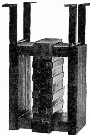
Fig. 240. Assembled Core Showing Method of Clamping
