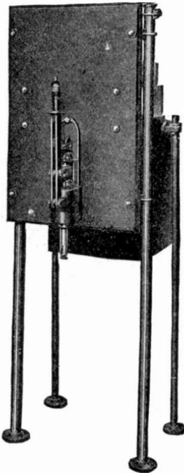
Fig. 383. General Electric Oil Break Switch Mounted on Panel
