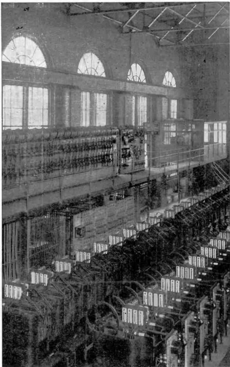
**GROUP OF FOUR-AMPERE SERIES RECTIFIER SETS AT PLUM STREET STATION, CINCINNATI, OHIO**
