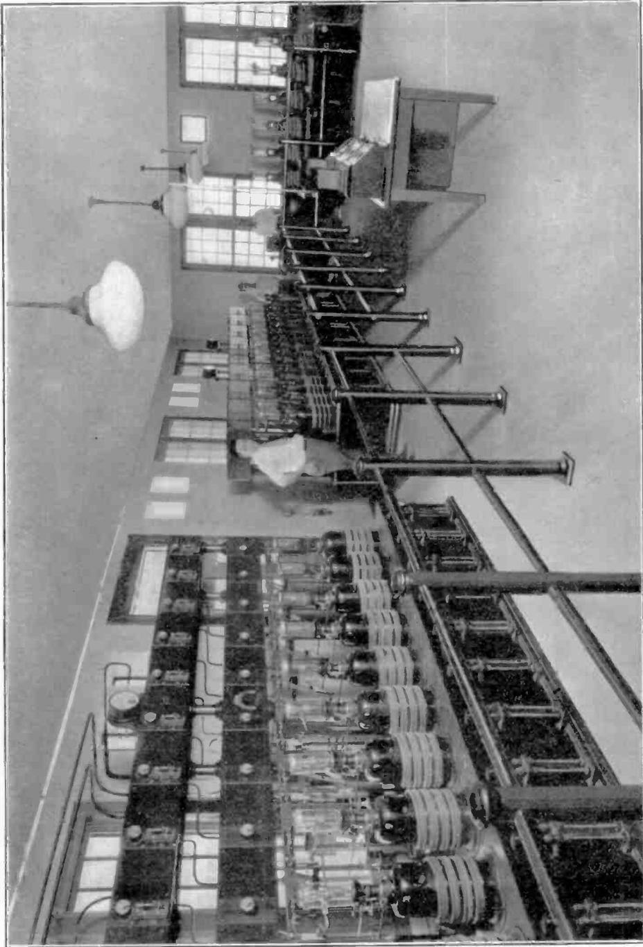
FIG. 38.—A general view of the thirty-two water-cooled tubes with which the WEAF transmitter of the National Broadcasting Company is equipped. Pure water from cooling tanks circulates through the coils of rubber hose at the base of the tubes. Each tube is equipped with a relay which drops and displays a small white disk in case of tube trouble.
