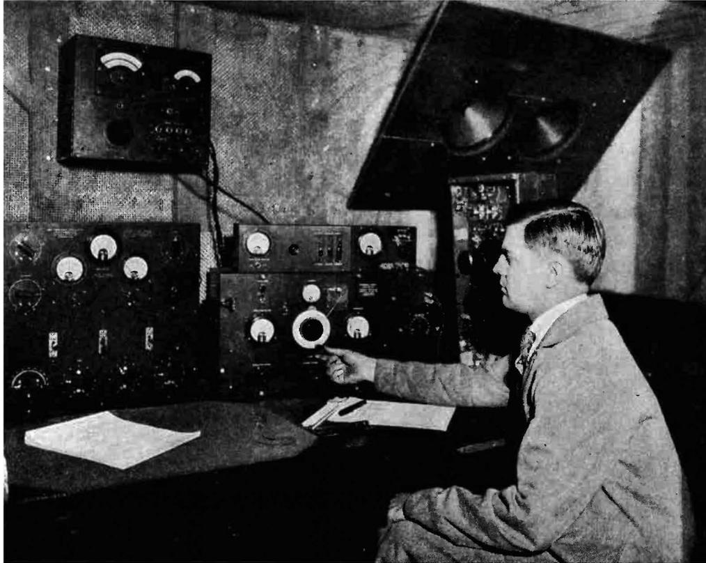
A SHIELDED ROOM IN WHICH RADIO RECEIVERS CAN BE TESTED FOR SENSITIVITY AND SELECTIVITY WITHOUT INTERFERENCE FROM NEARBY ELECTRICAL MACHINES AND CIRCUITS
