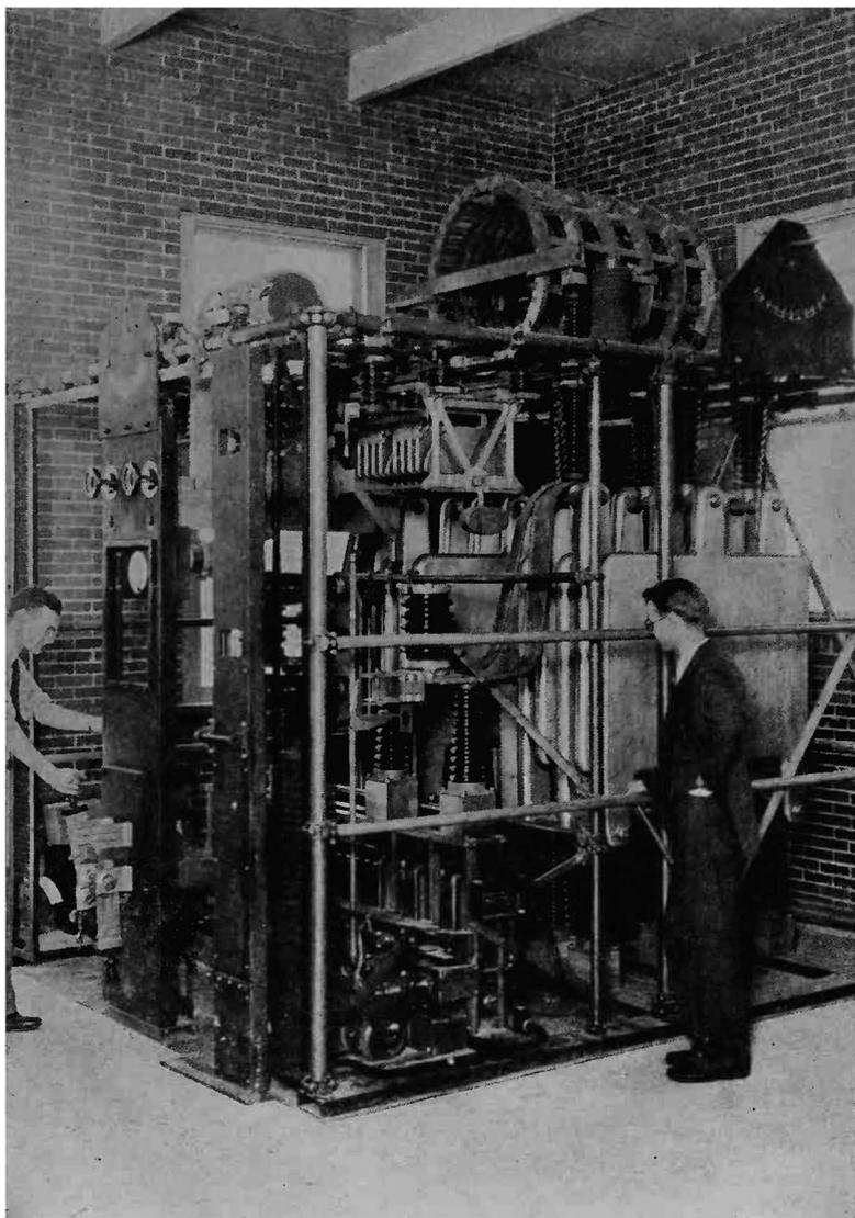
**HIGH VOLTAGE INDUCTANCE OR TUNING COIL AND CONDENSER LOCATED IN
