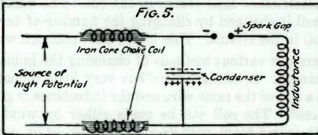
In order to have radio waves, the electrons must oscillate at the rate of 6,000 or more times a second. That is, to start a radio wave there must be an alternating current alternating at the rate of 6,000 or more times per second. Up until recent years, there was no generator built capable of producing alternations of so high a frequency. Only a very few such machines are in use to-day and those only at the very high-powered stations.
