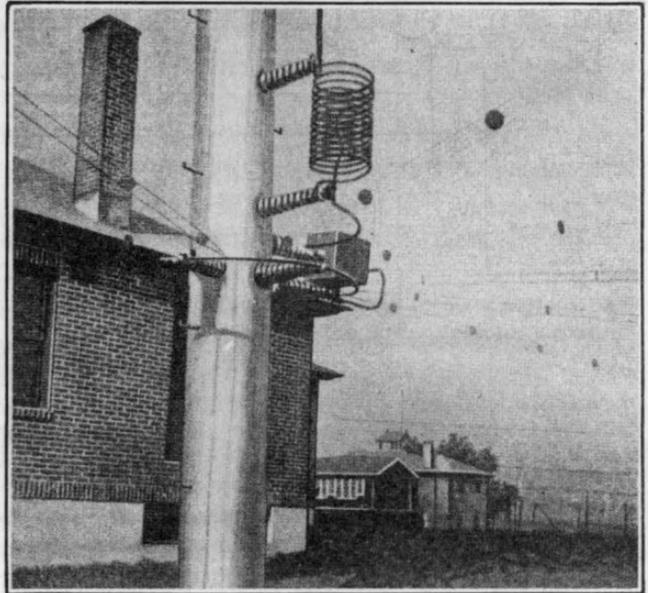
FIG. 284.—Antenna loading coil and ammeter—Station KDKA.
