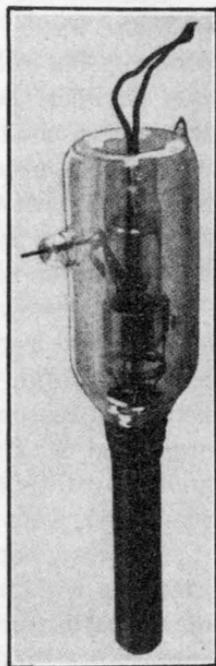
FIG. 179.—20-kilowatt water-cooled transmitting tube, type UV207.
