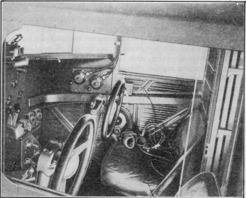
FIG. 466.—A view of the cockpit of a transport plane showing various components of the radio installation. Compare this illustration with the illustration in Fig. 452. *Courtesy Western Electric Company.*
