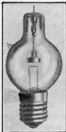
FIG. 76.—Tungar rectifying bulb.
