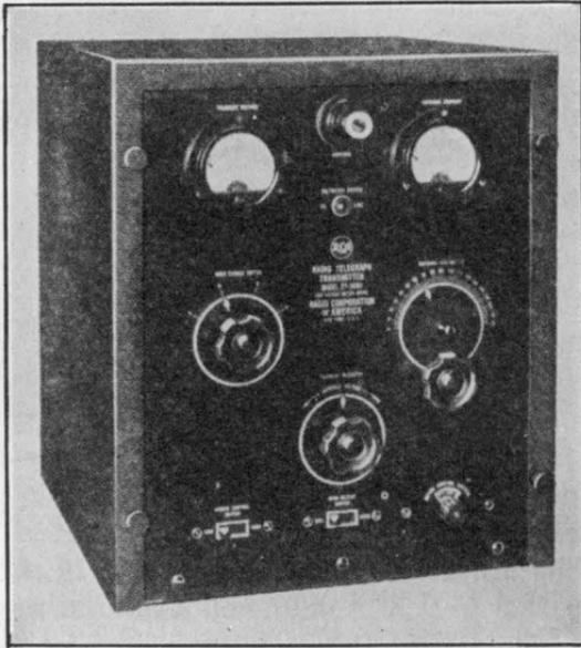
FIG. 367.—Front view of the type ET-3650 emergency telegraph transmitter.
