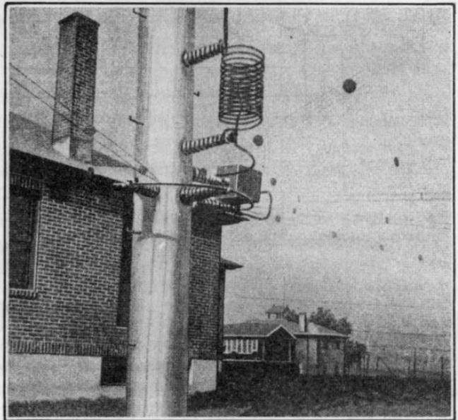
FIG. 284.—Antenna loading coil and ammeter—Station KDKA.
