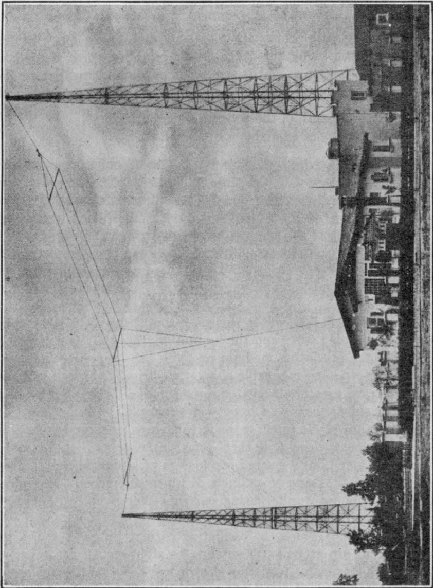
FIG. 274.—Illustrating "T" type antenna and supporting towers.
