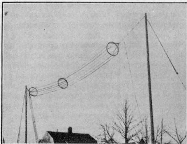
FIG. 277.—Cage type antenna with cage lead-in.
