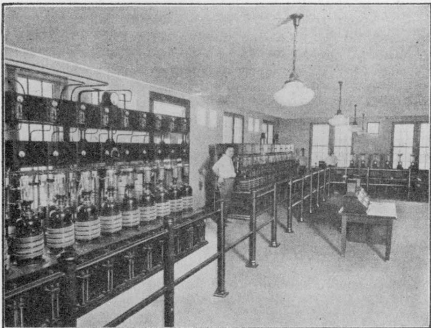
FIG. 322c.—A general view of the 32 water-cooled tubes with which the WEAFF transmitter at Bellmore, Long Island, N. Y., is equipped. The water circulates through the coils of rubber hose at the base of each tube. Each tube is equipped with a relay which drops and displays a small white disk in the case of tube trouble.
