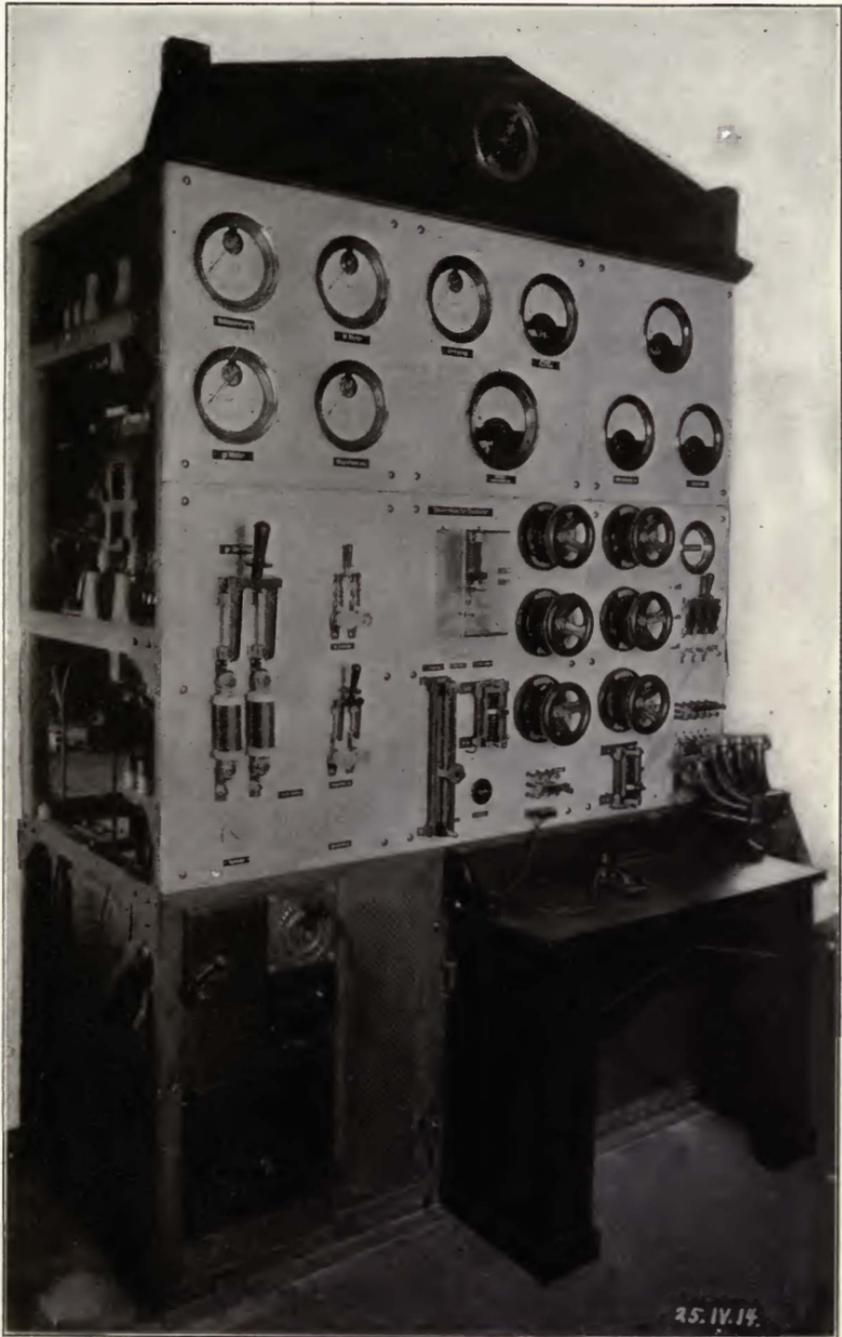
FIGURE 187—Telefunken Company 10 k.w. alternator-frequency doubler radiophone transmitter.
