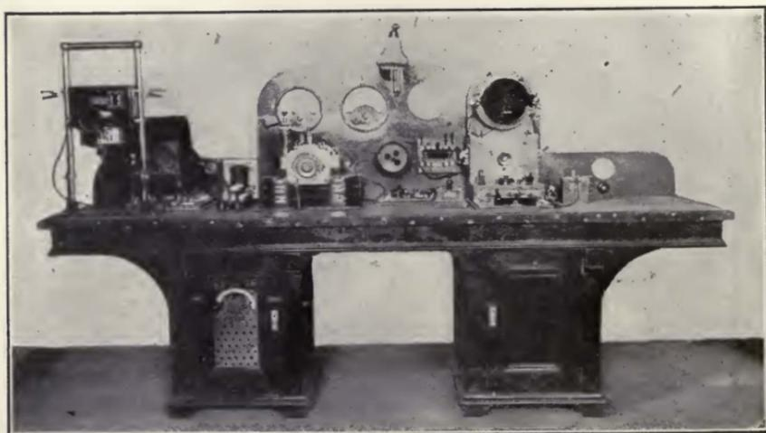
FIGURE 22—Berliner-Poulsen 3 k. w. arc radiophone station.
