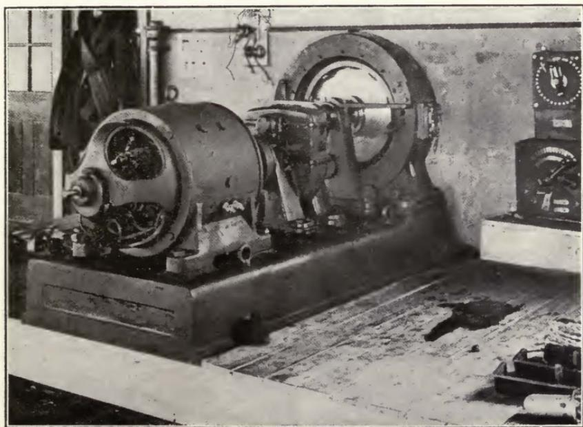
FIGURE 113—Telefunken Company 10 K. W., 10,000 cycle alternator.
