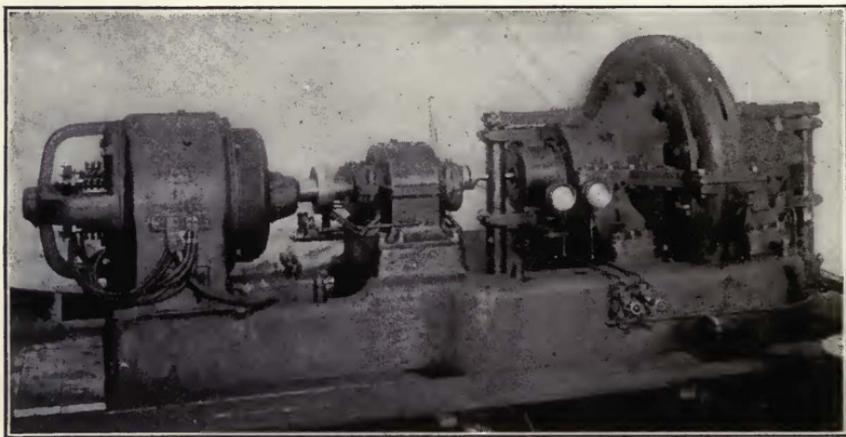
FIGURE 124—50 kilowatt, 50,000 cycle, General Electric Company-Alexanderson alternator.
