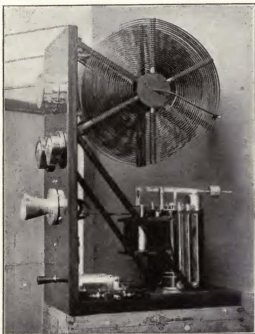
FIGURE 59—One-half kilowatt Hanscom radiophone transmitter.
