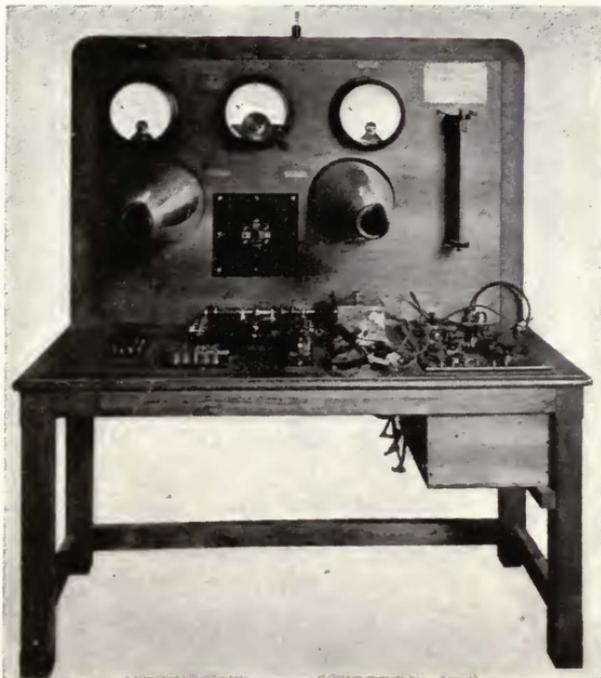
FIGURE 31—Colin and Jeance transmitting and receiving operator's table for radio telephony.
