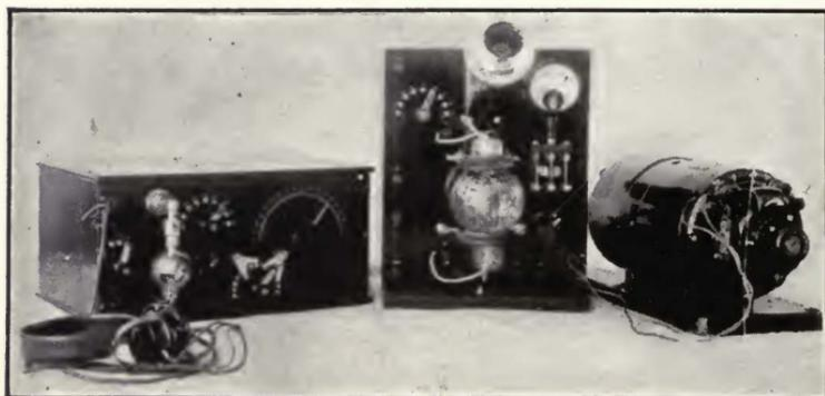
FIGURE 162—de Forest oscillion radiophone and radio telegraph transmitter and receiver (Type OJ3).
