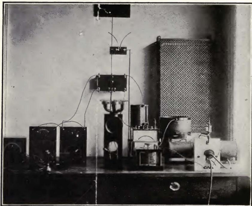
FIGURE 13—Danish Poulsen arc radiophone transmitter.
