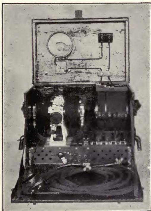
FIGURE 12—Berliner-Poulsen arc for portable stations.
