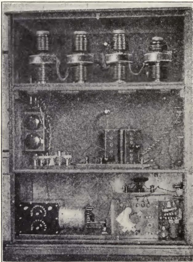
FIGURE 53—Ditcham radiophone transmitter and receiver.
