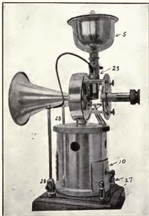
FIGURE 145—Scheidt-Boon Marzi high current microphone transmitter (relay type).
