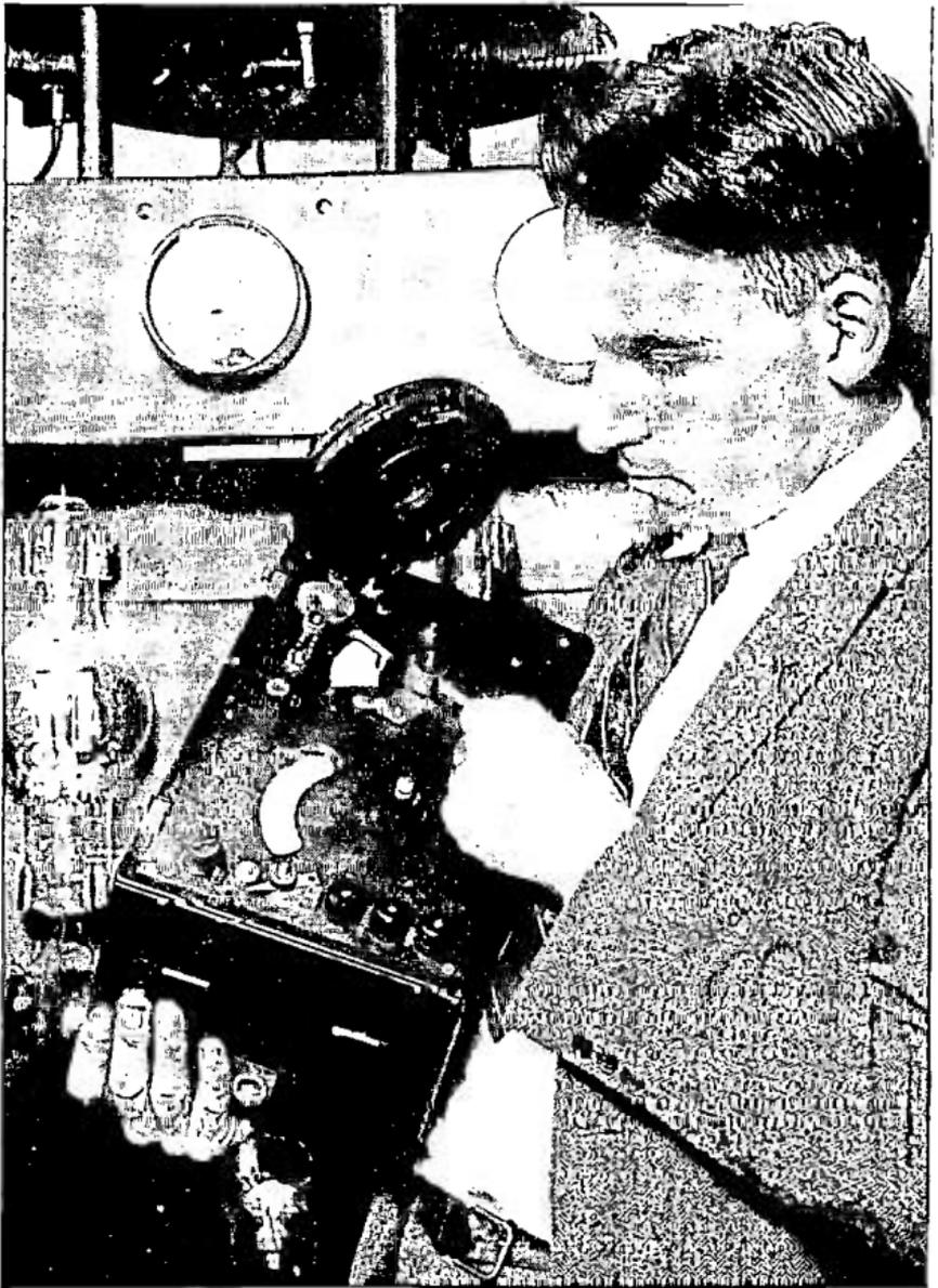
ADJUSTING WAVE LENGTHS WITH A WAVE METER
