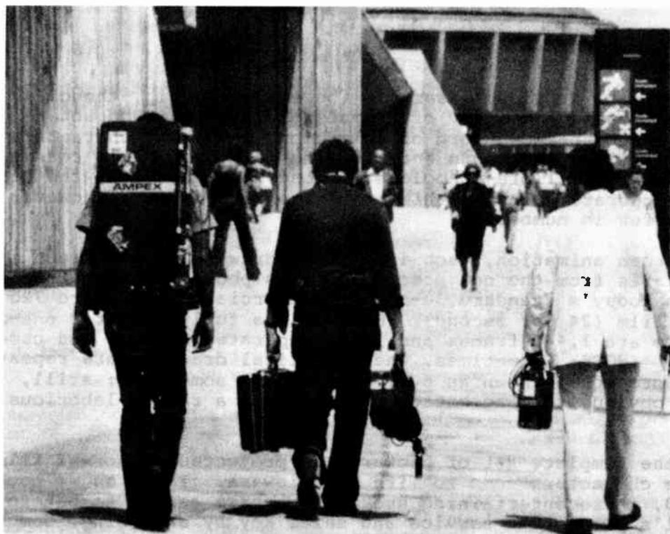
**Fig. 11.6.** Ampex VR-3000 portable videotape recorder, mounted on a backpack frame. (Courtesy of Ampex Corporation)
