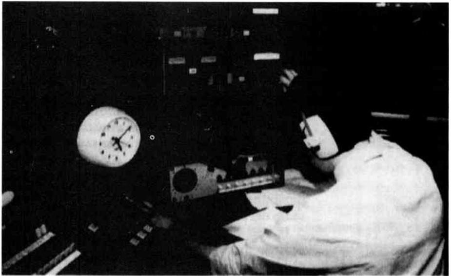
**Figure 59** Newsbooths are designed so reporters can present their own news programmes without technical assistance. Peter Heaton-Jones operates a simple mixing panel (left) while reading the cue to an interview. The moment he finishes the cue, his right hand will fire the cart containing the interview. The big meter in the centre of the stack helps him adjust the levels (Andrew Boyd)
