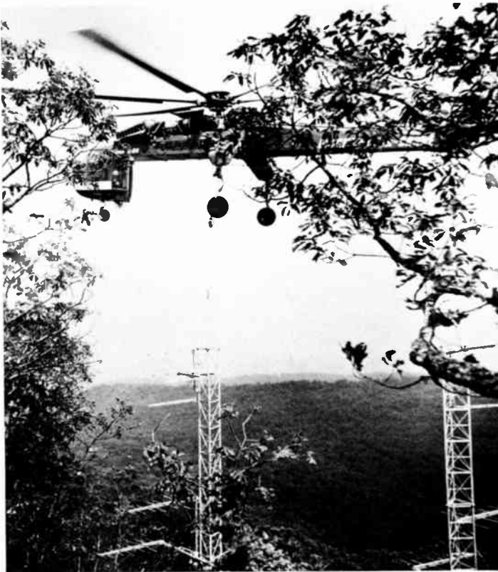
Figure 6-3 Critical to the effective operation of the cable system is the master antenna. Often located on mountain tops and in rough terrain, constructing the antenna can be dangerous and expensive. (NCTA)
