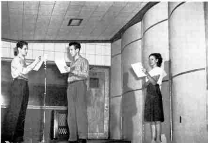
10. Pylon Construction. Here is a corner of Classroom Studio A at the University of Oklahoma. Notice the vertical pylons and dropped ceiling.
