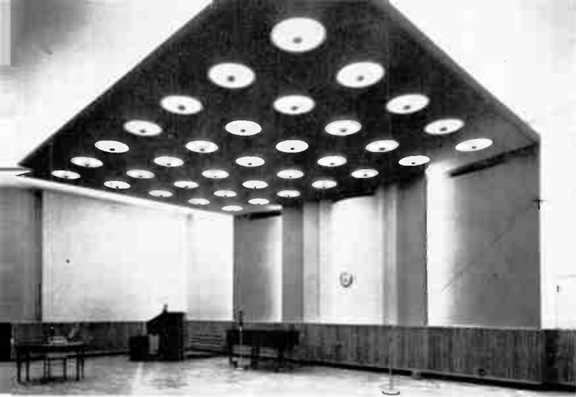
9. Dual AM-TV Studio, 33' × 45'. Two Stories High. It can be adapted for either radio or TV productions; walls include "splayed wing, as well as cylindrical reflectors. Resilient, squeakless floor is made by 1' lengths of tongue-and-groove beech, fitted and held in place by mastic. An acoustical canopy is suspended above the work area. (Photo by courtesy of WGN, Chicago.)
