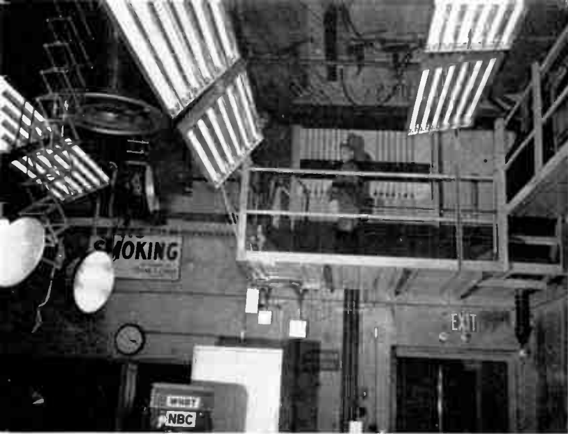
28. Lighting Crew at Control Switches. Lighting is controlled from central switchboard at WNBT. (Photo by courtesy of the National Broadcasting Company.)
