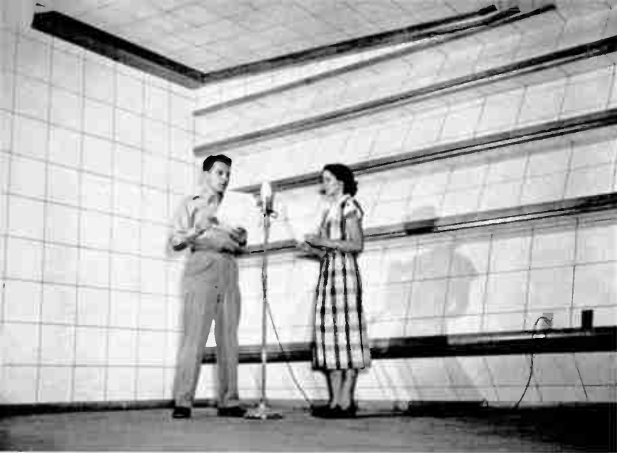
11. Saw-Tooth Wall Construction for Extreme Acoustic Deadening.
