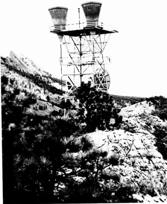
FIGURE 7-1 Microwave antennas, such as these near Boulder, Colorado, provide long-distance communication without wires. Microwave systems are especially efficient in areas which are too remote to economically construct wired systems. (AT&T)
