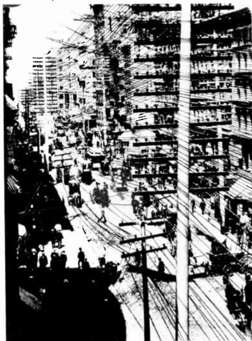
FIGURE 2-7 The early prosperity of the telephone industry is graphically illustrated in this picture of telephone wires strung in New York City in the 1880s. By the late 1880s, the Bell Telephone Company had been formed, lines were into New England, and substantial progress had been made linking telephone companies in the Midwest. (Photo Courtesy Western Electric Company)
