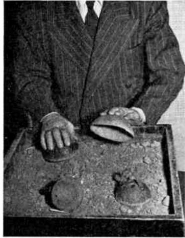
Fig. 26. Since a horse cannot be brought into the studio, the technician must resort to synthetic means to achieve the sound of hoof beats. (Courtesy CBS)
