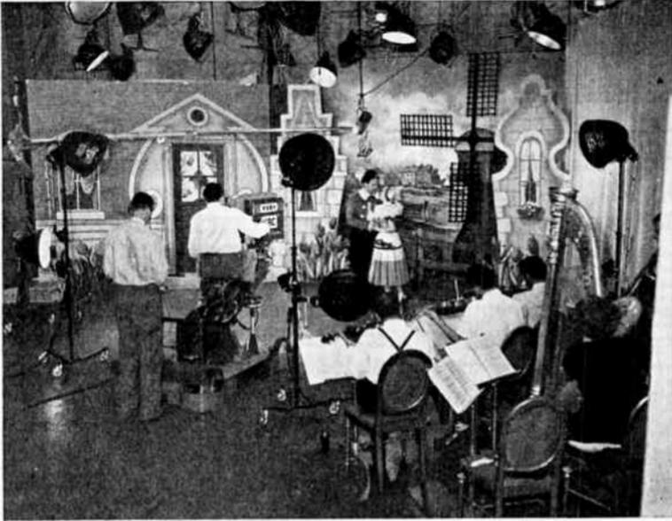
Fig. 35. A TV-studio scene. Note the floor manager behind the cameramen, the carriage or 'dolly' permitting the camera to be rolled around, the microphone-boom man at the far left, and the two sets side by side. (Courtesy NBC)
