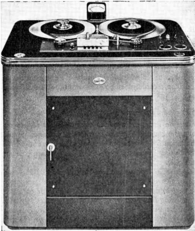
Fig. 21. A magnetic tape recorder that can record up to two hours of programs. (Courtesy Presto Corp.)
