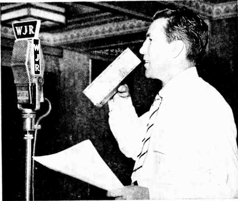
FIG. 29.—Actor using a muffle box, which is a cigar box with a half-moon cut out of the end, to create the effect of a person speaking from behind a closed door or of an off-stage voice.
