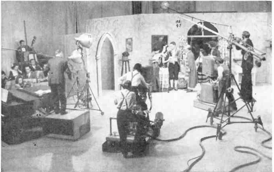
FIG. 38. This photograph in the studio of WRGB shows how compactly the actors are grouped. To the left is the orchestra for musical interludes and background. In the immediate foreground is a camera on a dolly; another camera is to the right; and the microphone boom to the extreme right is hung above the actors. ( General Electric—WRGB. )
