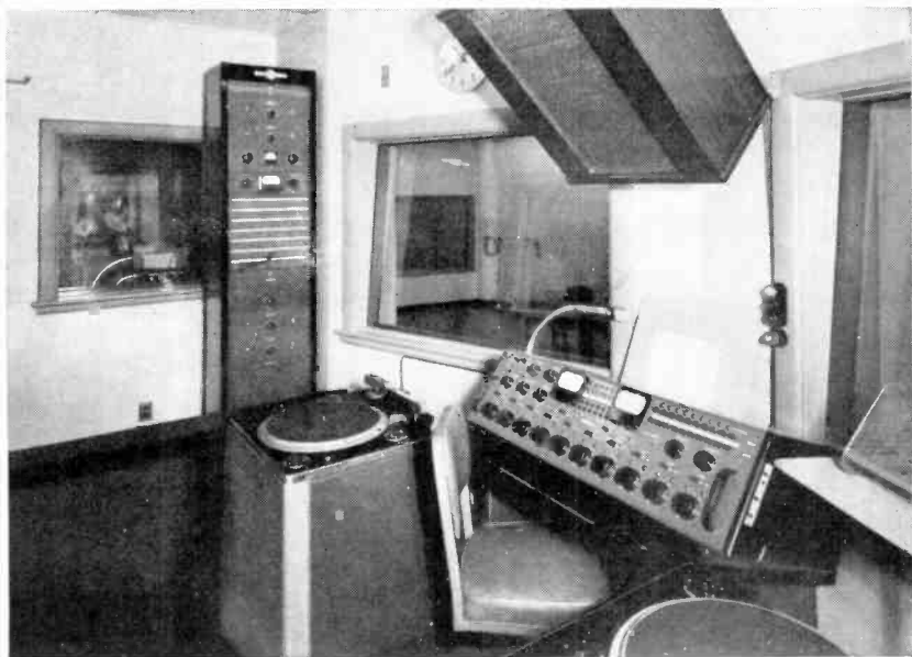
FIG. 14. Control console and rack, Station WUOM (Collins Radio). This control room serves two studios. WUOM has no master control. ( University of Michigan. )
