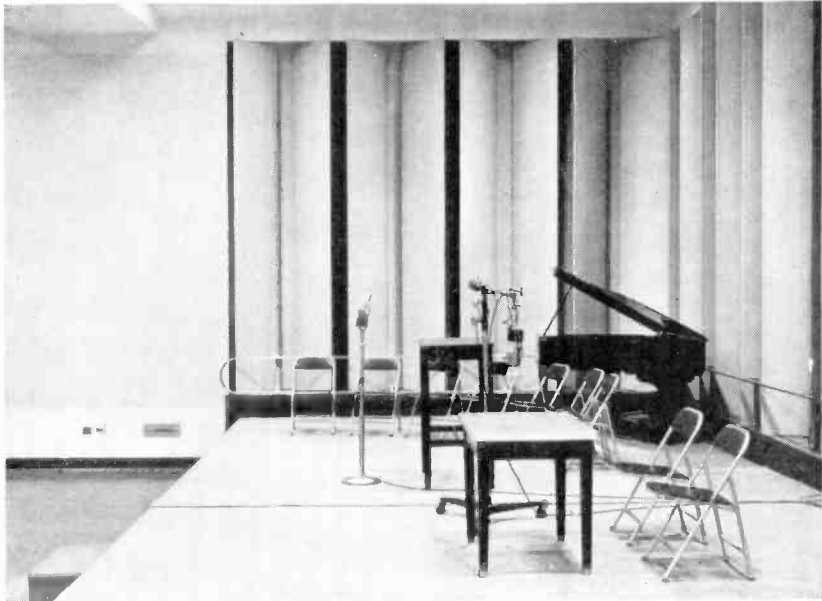
FIG. 2. Revolving acoustic walls, C.B.S. These panels open and are reversed to liven or deaden the studio as required. ( Columbia Broadcasting System. )
