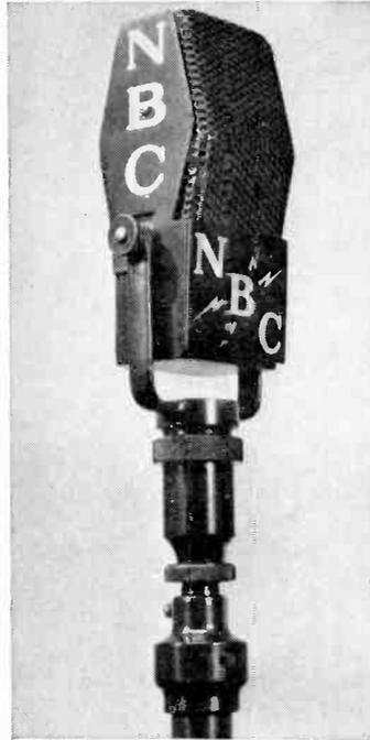
FIG. 3. Bidirectional velocity or ribbon microphone. (R.C.A.)
