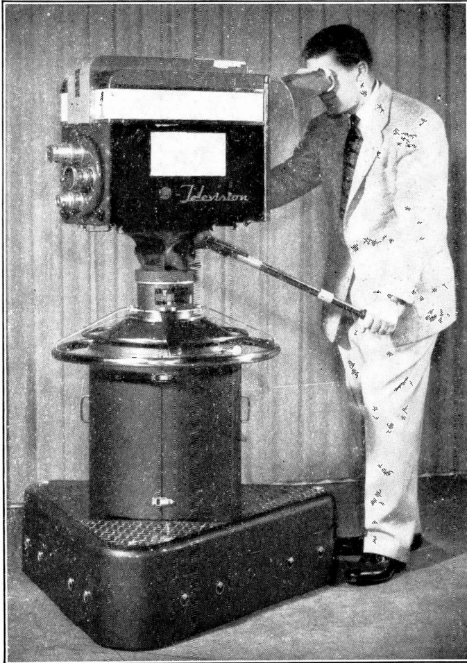
FIG. 74. The PD-3 pedestal and the friction head mount.
