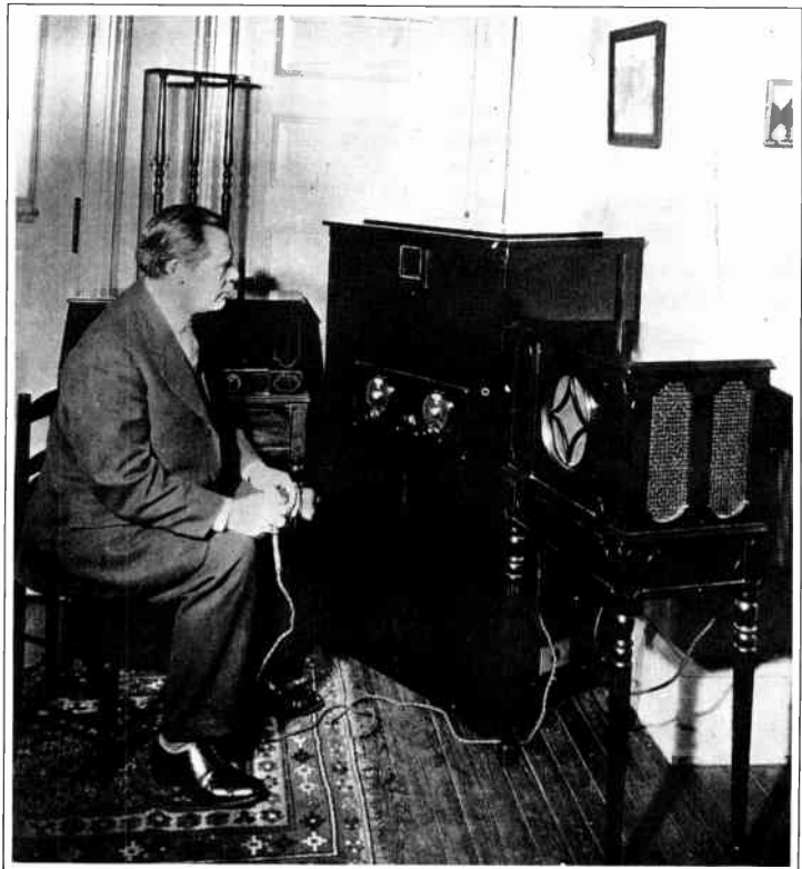
An early experimental TV set with a screen not much larger than a pack of playing cards. All three pieces of equipment were needed for the receiver.
