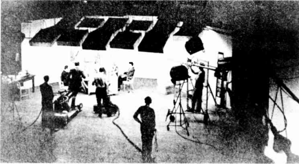
Figure 4.8 CBS 1940s television studio. Technicians felt that early TV cameras needed an even wash of bright light to make good pictures. Incandescent lights would make a studio unbearably hot, so some pioneer television production facilities were equipped with banks of fluorescent lights, as was this CBS studio. After the wash was established, spotlights beamed in additional light to give the effect of highlighting. (Source: William C. Eddy, Television: The Eyes of Tomorrow . New York: Prentice, 1945. Used by permission.)
