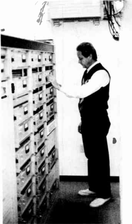
Figure 12.22 Cable system headend. A technician adjusts a control at Cox Cable-University City's headend. At left is the front of one rack of equipment; at right, the back of another—two of many that fill the small cement-block building. All signals feed to the box at top, the first amplifier in the system. From the other side of the amplifier emerges the trunk line, which carries programming throughout the franchise area.
