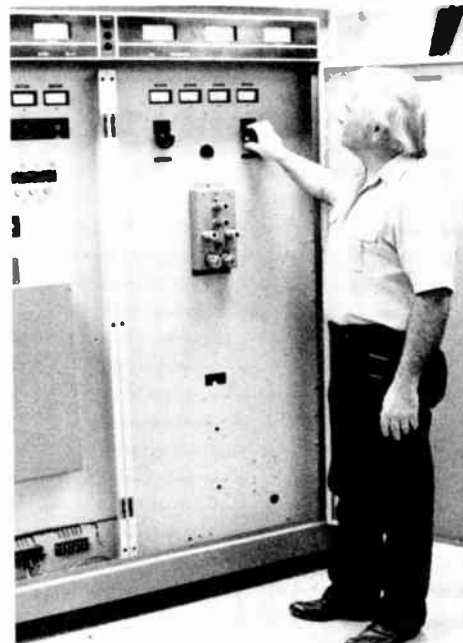
Figure 19.2 Radio station transmitter room. WRVF Chief Engineer Ed Slimak adjusts the transmitter.
