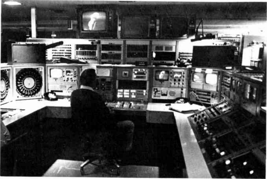
Figure 4-21 The television control area is the hub of studio activity where an engineer not only can control live programming, but monitor and switch network feeds and, in some stations, direct in-house editing and production. (WRTV)
