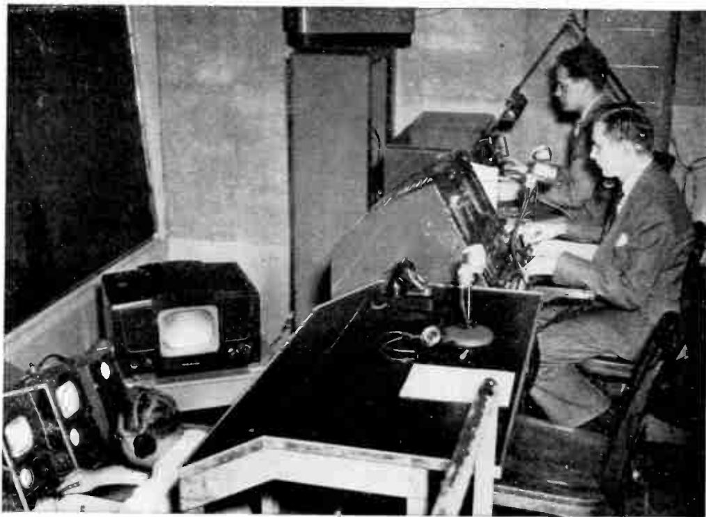
Control room, WPIX, New York. Video engineer, bottom left, director's chair, technical director and audio engineer, at right
