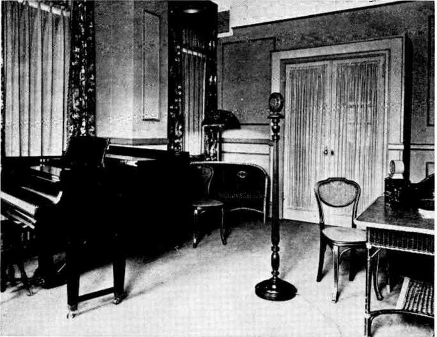
FIGURE 46. *Studio of about 1930. The heavy drapes had disappeared because microphones had been improved and the studios were better designed acoustically. (Courtesy of National Broadcasting Company.)*
