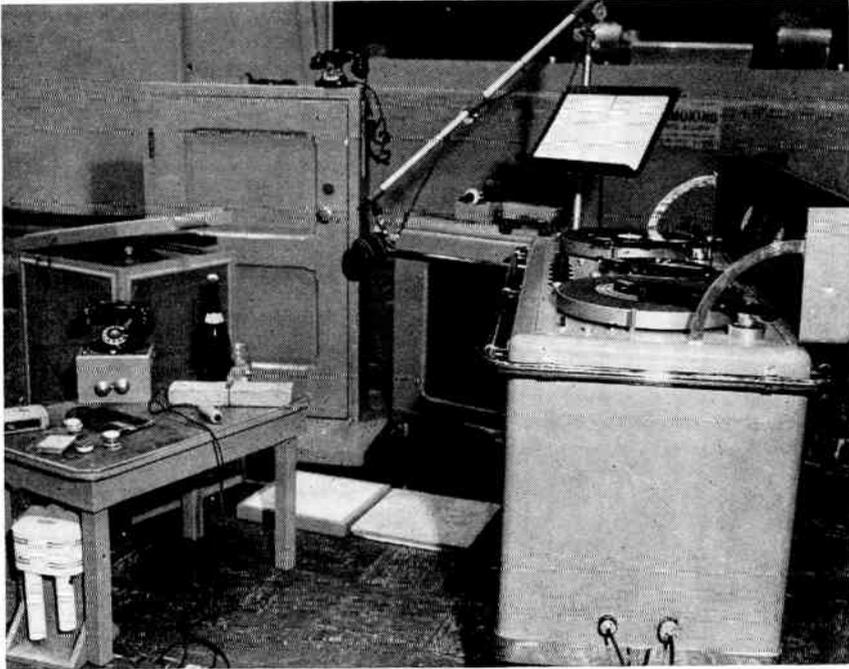
FIGURE 23. *Sound setup for one soundman showing placement of cardioid mike. (Courtesy of Don Lee Broadcasting System.)*
