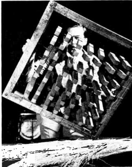
FIGURE 11. A manually operated device to secure the sound of marching feet. The suspended wooden pegs are rhythmically dropped on the broom corn. (Courtesy of the National Broadcasting Company.)
