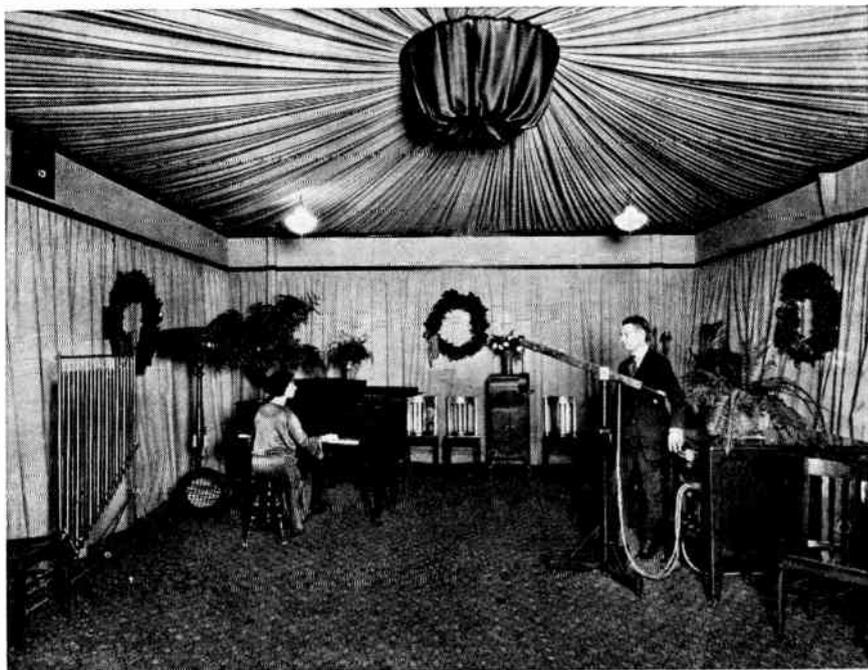
FIGURE 40. *The first "designed" studio at KDKA was installed in 1922 after the tent studio on the roof had blown away in a heavy wind. The draped ceiling and walls cut down room resonance. (Courtesy of Westinghouse.)*
