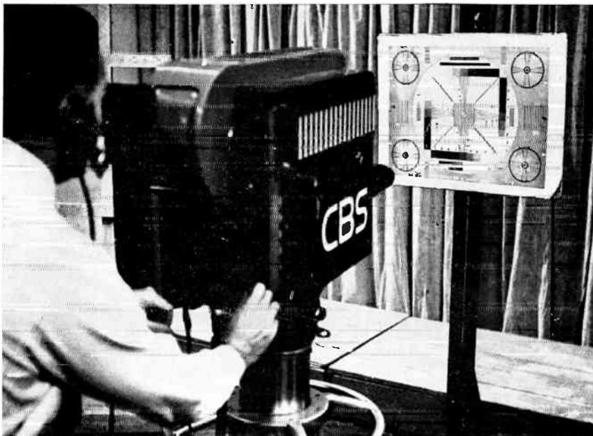
Fig. 3-3. Cameraman lining up on test chart.
