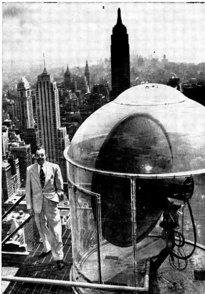
Fig. 20-5. Plastic Radome protects microwave receiver atop Radio City from wind and weather.
