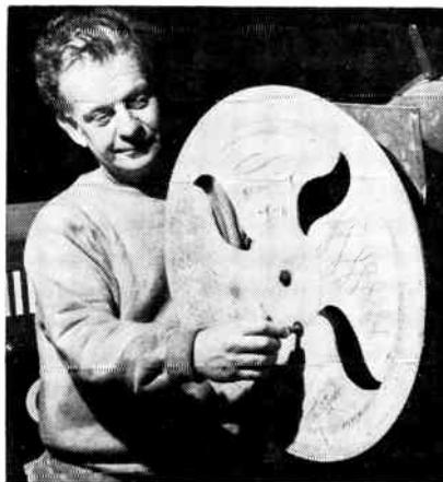
Fig. 18-22. Gloccamorra for firelight or other uneven or flashing light.
