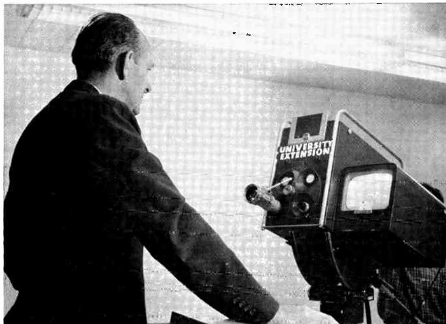
Fig. 22-1. The camera with the picture on the front. This production aid, devised by the author, provides the TV performer with constant knowledge of the program without taking his eyes from the viewing audience.
