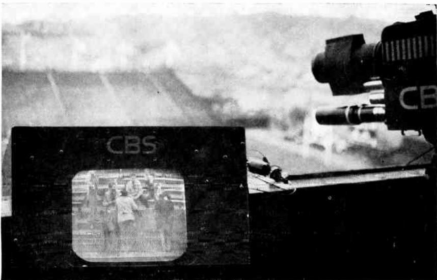
Fig. 5-5. Video Reflectar lens (early model) focused on people in the stands across a football field. The camera's picture is visible on the monitor in the foreground.
