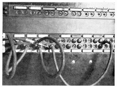
FIG. 53.—A coaxial-cable jackboard connecting studio and apparatus.
