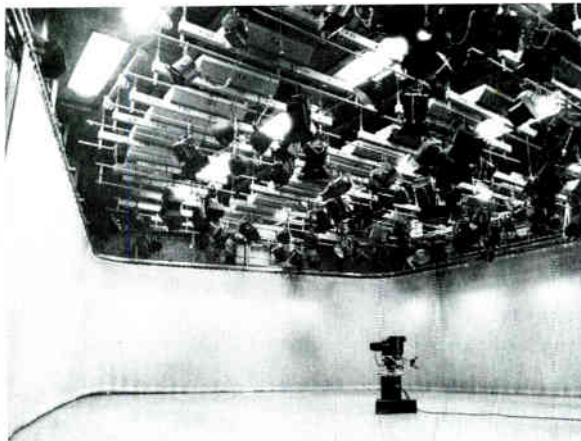
12·46 The cyclorama provides an ideal background for a great number of productions, especially for open-set designs.
