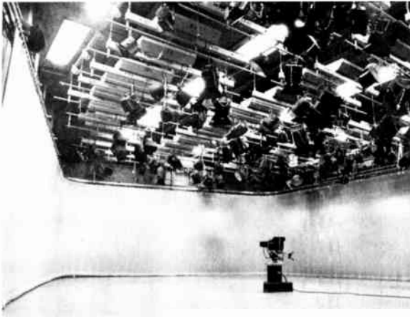
12-46 The cyclorama provides an ideal background for a great number of productions, especially for open-set designs.
