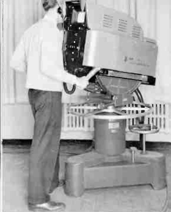
Figure 18. Color Orthicon Camera, RCA TK 41, on Cradle Rocker.
