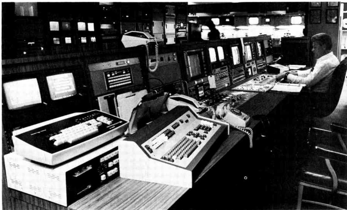
Fig. 3-7. The master control room of a medium-sized television station. Photo by Greg Wright. (Courtesy WHIO-TV)
