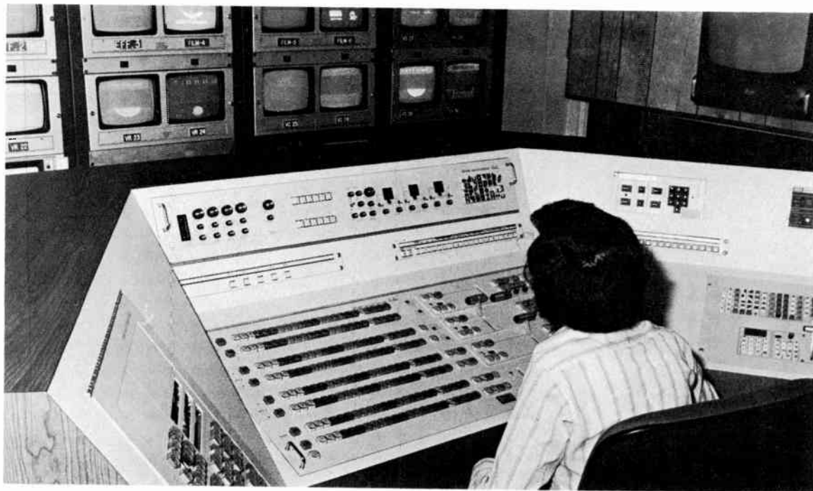
Fig. 4-7. A technician and the Grass Valley Switcher, which manipulates all video sources during a production session. Photo by Greg Wright. (Courtesy WHIO-TV)
