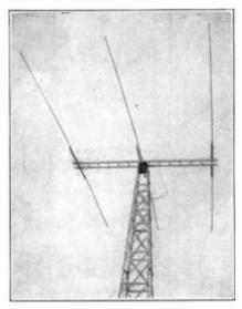
Figure 15. TYPICAL INSTALLATION OF 3-ELEMENT CLOSE-SPACED ARRAY.
