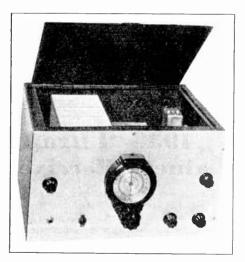
Figure 15—The 1938 "Ultra Gainer" receiver, showing fully enclosed coll shield compartment and front panel layout.
