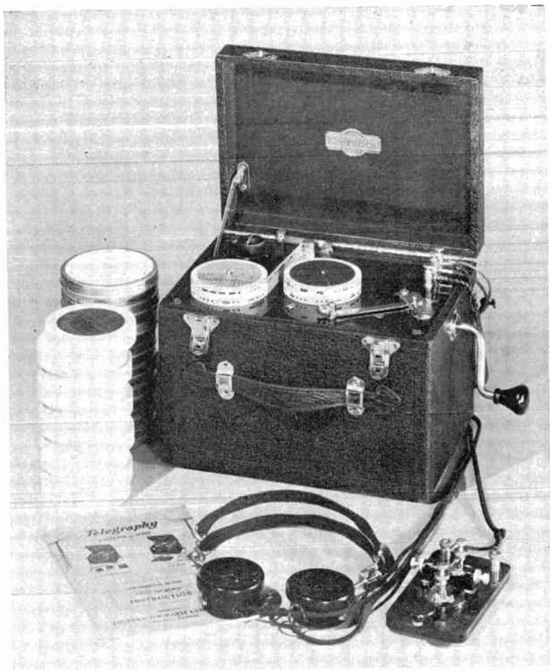
102. The Instructograph machine for teaching the sending and receiving of telegraph code. ( The Instructograph Company. )
