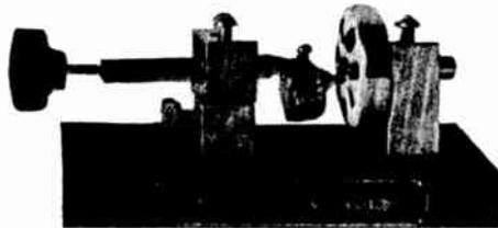
Two early crystal detectors. The contact point could be adjusted or changed to find the most receptive spot on the crystal.
